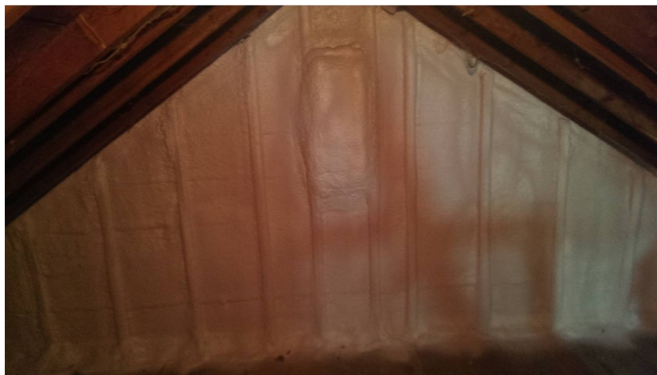
Figure 15. Interior-applied foam on the gable end
