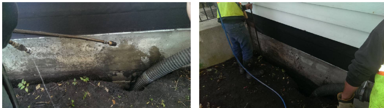
Figure 6. The hydro-vac high-pressure water wand and vacuum used to create the trench
