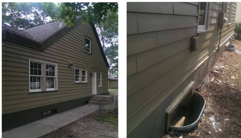
Figure 12. Completed foundation insulation with trim and windows
