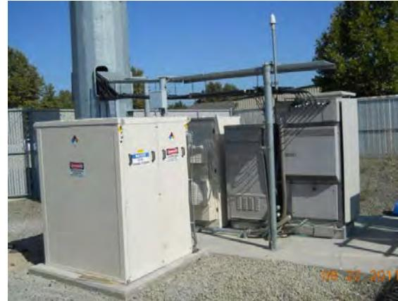
These units can be configured to provide a full 72 hours of backup power for many different types of cellular tower sites.
