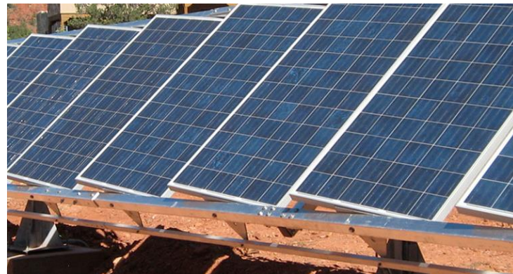
Low-cost, coarse 2-axis tracking with high acceptance angle and flat external surface
