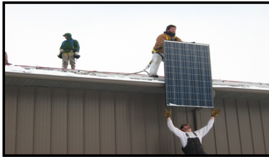
Figure 2 Solid Waste Building
