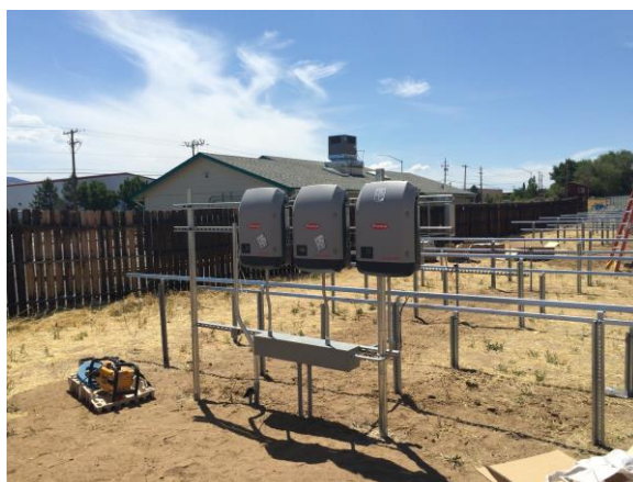
Installation of electrical components box
