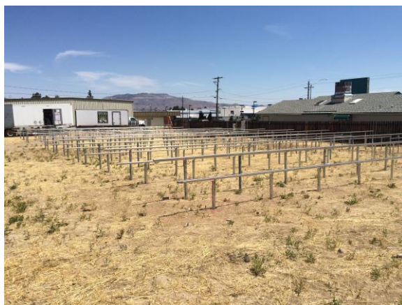
Installation of post and racking system
