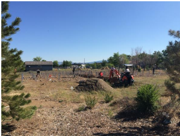
Trench excavation and post installation
