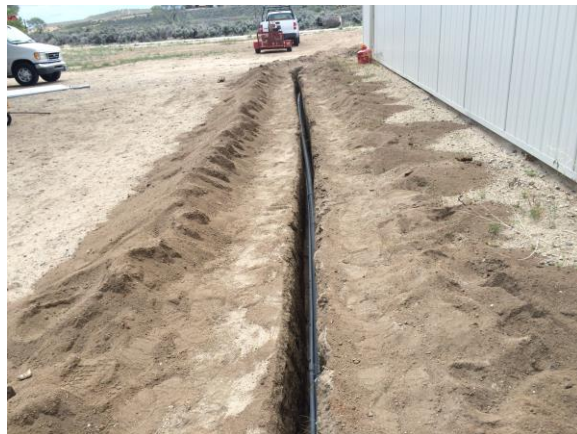
Trenching and laying wire
