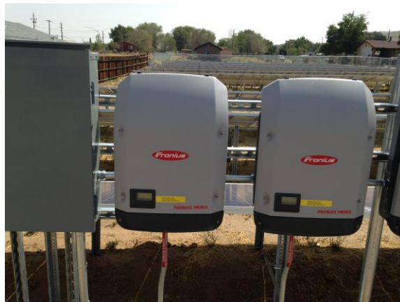
Installed inverter box and electrical components
