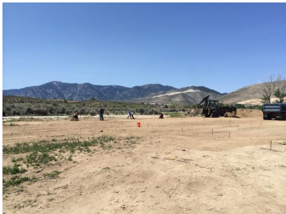
Site grading and staking
