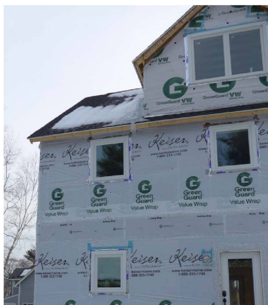
Figure 6. A later BrightBuilt Home in which house wrap was installed outside of the foam insulation
