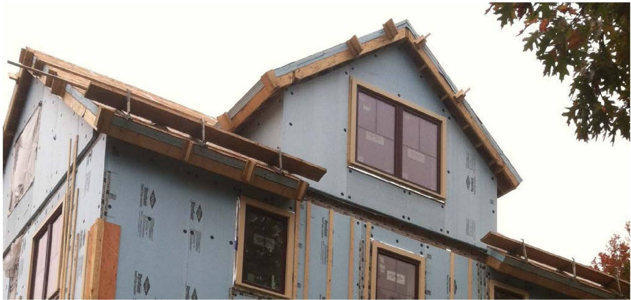
Figure 10. Four inches of XPS were installed above the first roof deck. A second deck, paper, and asphalt roofing were installed above the foam.
