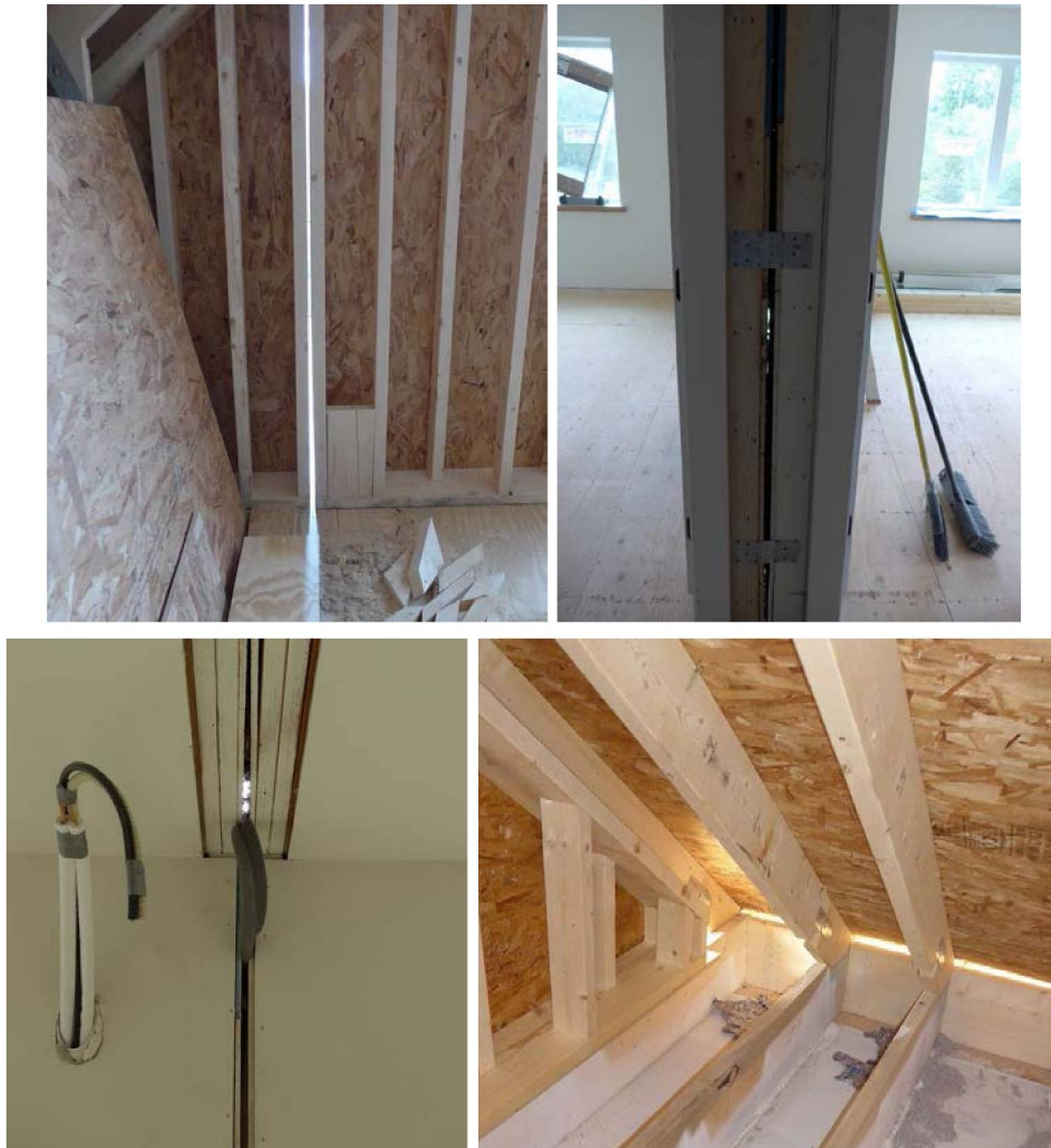
Figure 11. Gaps soon after set. Clockwise from top left: large gap in gable wall; daylight seen through marriage wall between bedrooms; damaged gasket between boxes on first floor; gaps at tilt-up roof.
