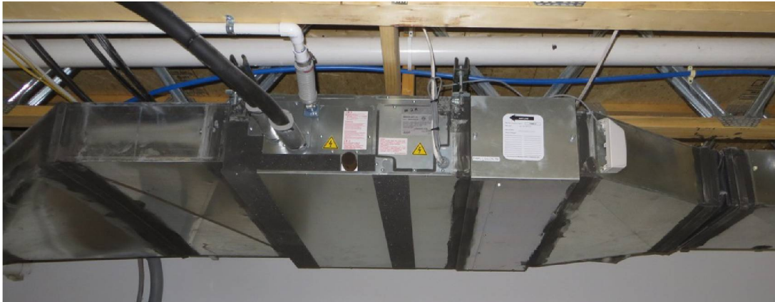
Figure 14. A “slim” ducted heat pump fan coil
