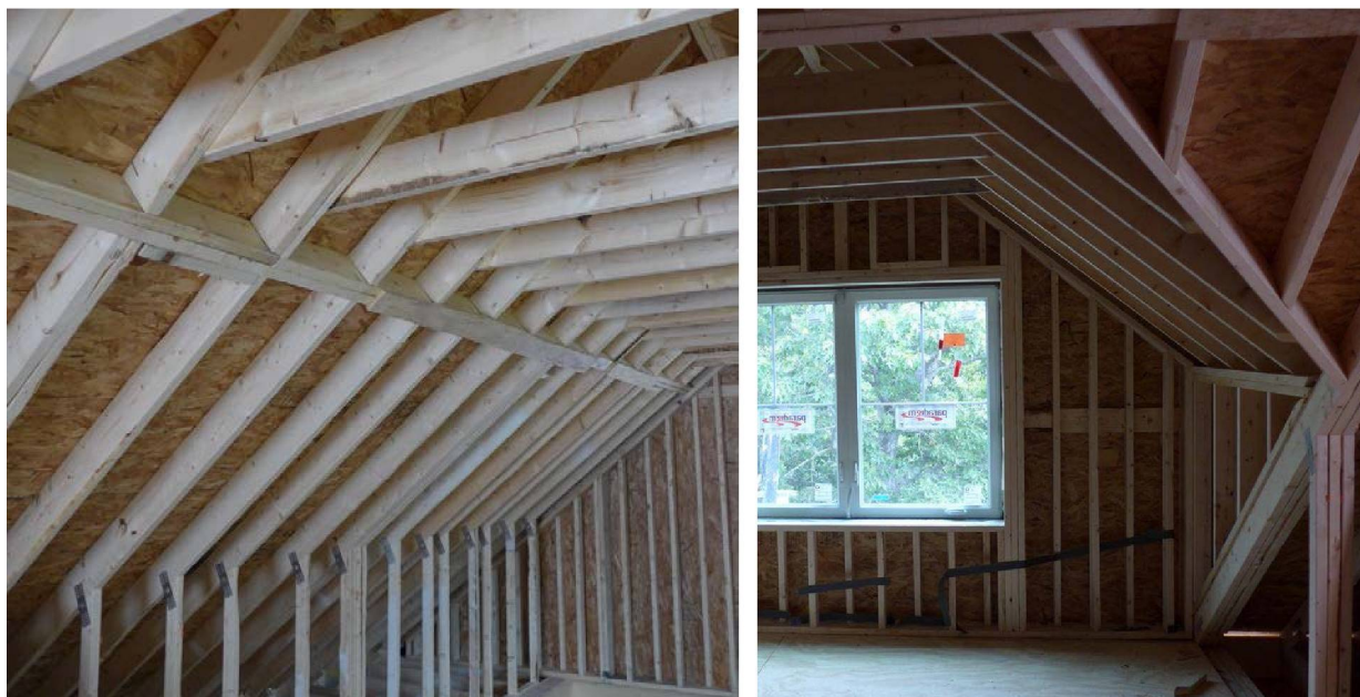
Figure 9. The tilt-up roof (left) and factory-assembled dormer (right)
