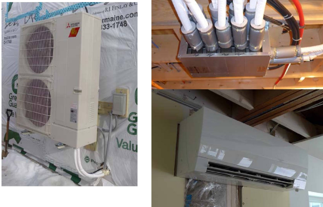
Figure 13. The heat pump outdoor unit in this BBH home under construction connects through a branch box to five ductless fan coils.
