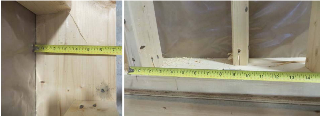
Figure 3. A 2x8 bottom plate with staggered 2x4 studs in the factory. The gypsum board is visible through the vapor retarder.
