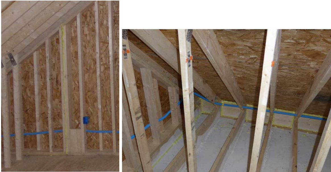
Figure 12. Gable wall and roof gaps appeared well sealed with foam and blocking.
