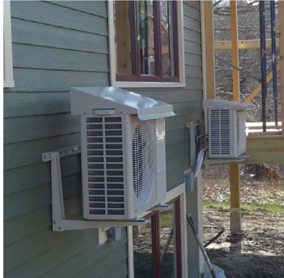
Figure 15. To ensure better winter performance, heat pumps are located well above snow level and covered to protect them from snow and ice.
