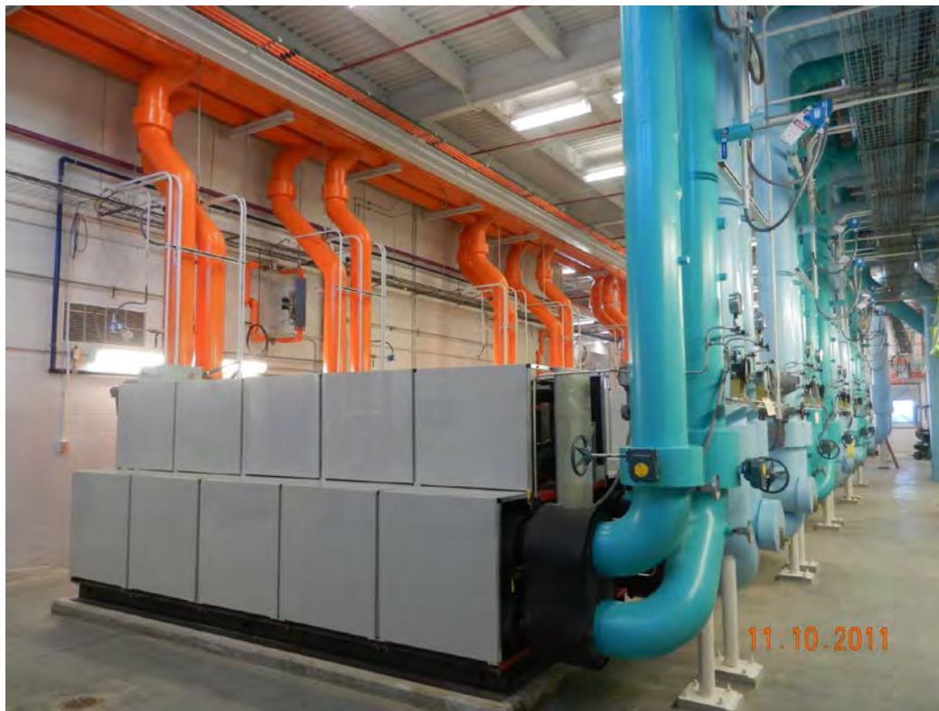
Photo 6: 10 Stage Heat Pump Bank
