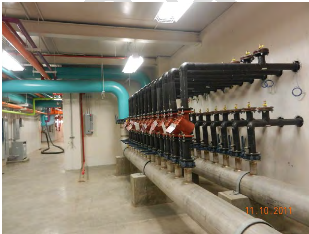
Photo 4: Well Field Pipe Header system in plant basement.
