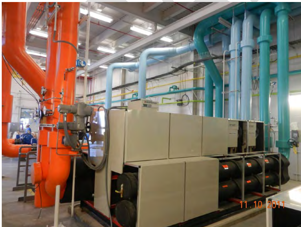
Photo 6: 10 Stage Heat Pump Bank
