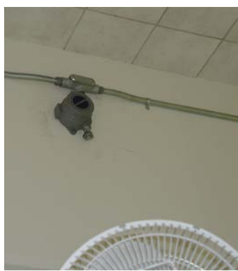
Hydrogen sensor mounted near a ceiling, where gaseous hydrogen is most likely to concentrate.
