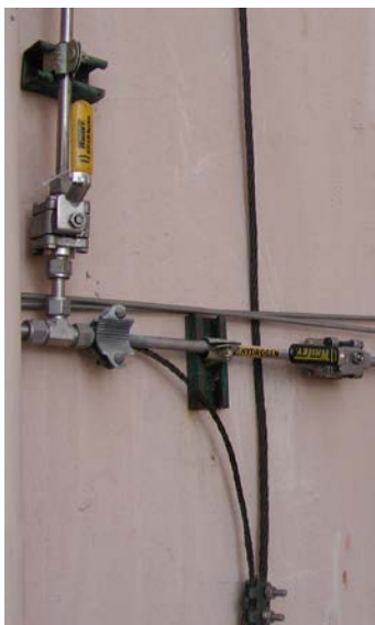
Grounding a hydrogen system.
