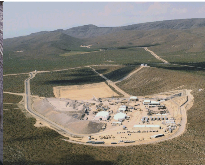
Aerial view of ESF surface facilities; north and south portals
