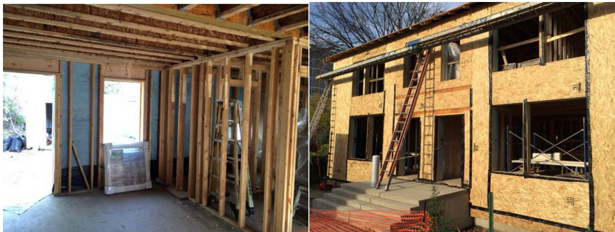
Figure 9. Wall construction—the 2 × 6 frame wall with air barrier membrane (blue) visible (left); the SIPs installed (right)
