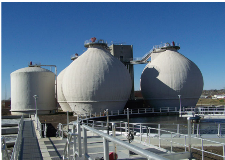
Figure 38. Anaerobic digesters at a wastewater treatment facility
