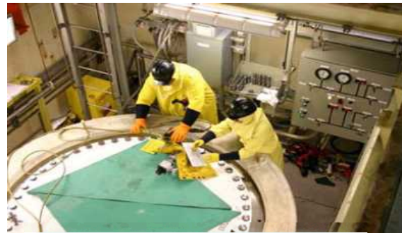
Lid Installation of a TN-32 Cask
