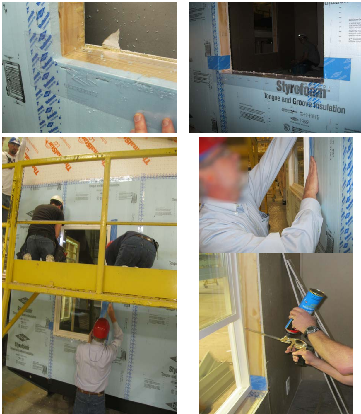
Figure 3. Window flashing system in House C
