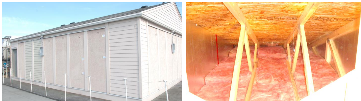
Figure 19: Coquitlam test facility (left) and vented attic (right)
