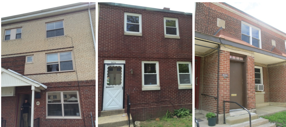
Figure 11. Typical PHIHA dwelling unit exteriors
