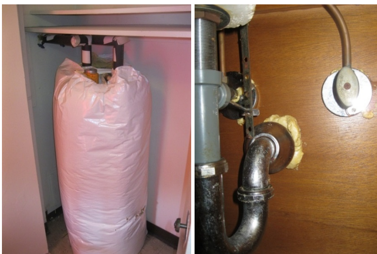
Figure 3. Electric storage water tank with insulation wrap (left); foamed plumbing penetrations (right) at IHA
