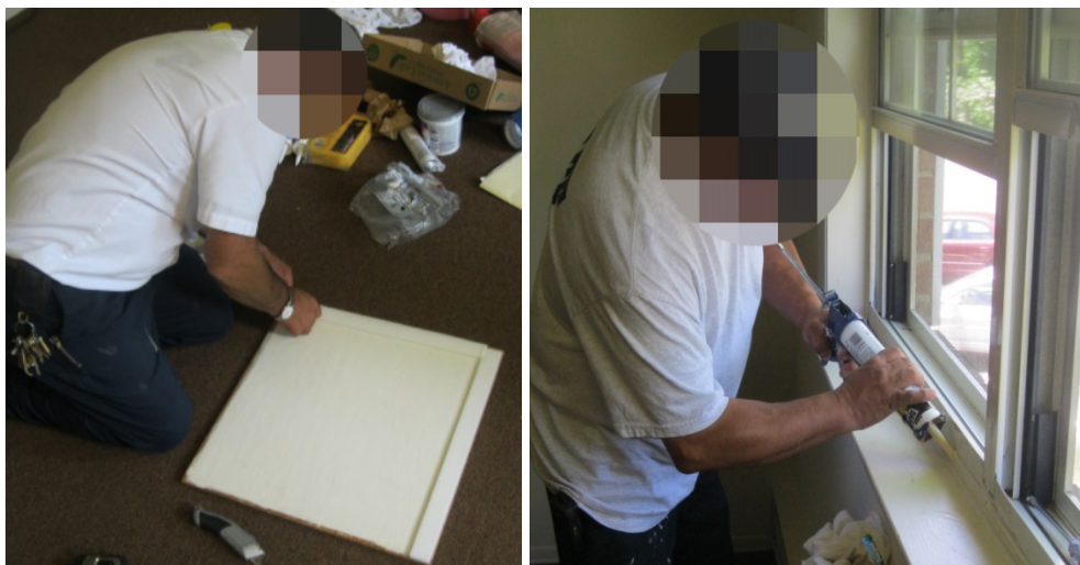
Figure 4. Installing gasket on attic hatch (left); caulking gap around window (right) at IHA
