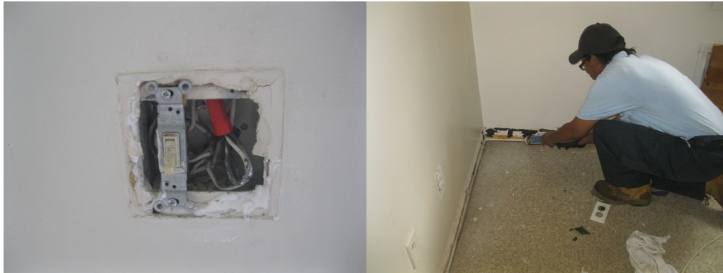
Figure 16. Newly caulked electrical outlet (left); caulking around base molding (right) at NHA
