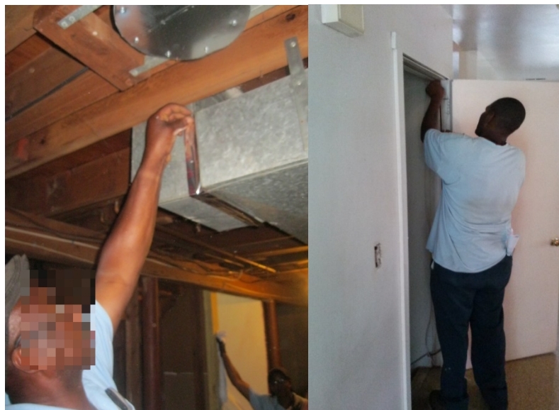
Figure 17. Sealing ductwork with Underwriters Laboratories-181 tape (left); installing weather stripping on door to unconditioned basement (right) at NHA
