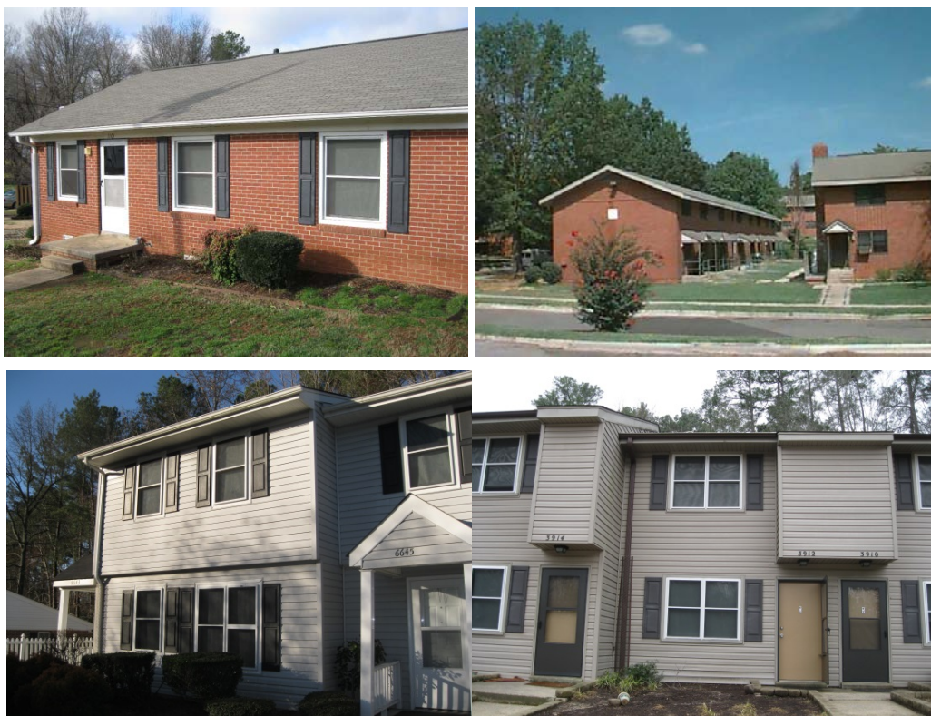
Figure 7. Typical RHA housing units
