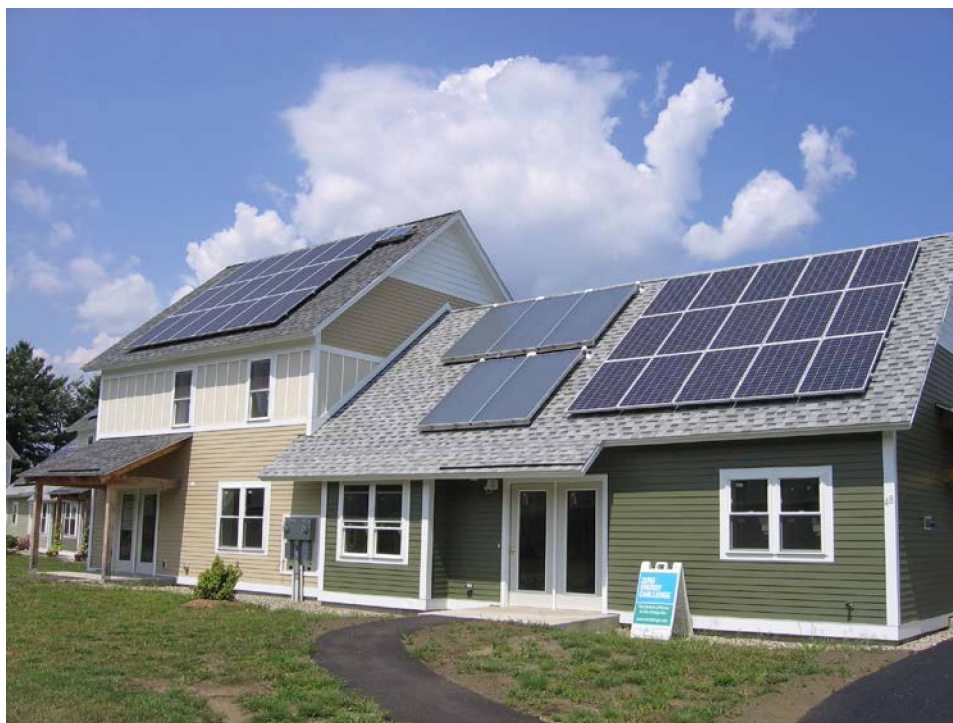
Figure 3. One of the duplexes at WWSV
