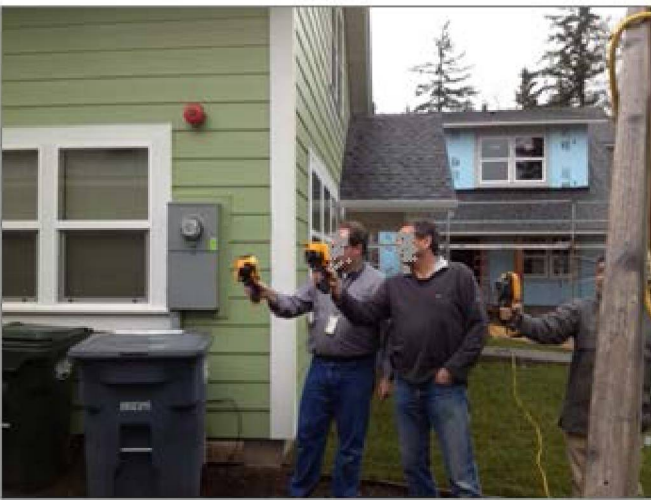
Fluke staff training HFH QA staff in the use of IR thermography to locate air leaks and insulation voids.
