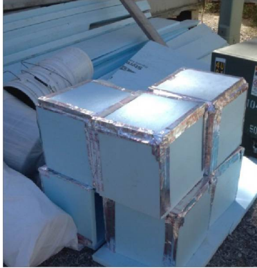
Insulated box for fire-suppression sprinklers used to help seal and separate from loose fill attic insulation
