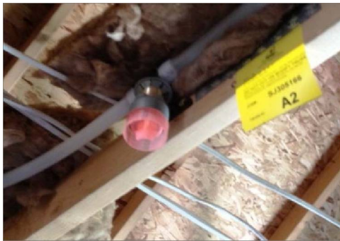
Sprinkler rough install
