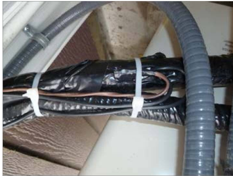
Figure 9. Vapor line thermistor
