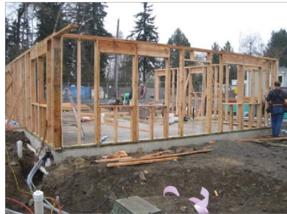
Figure 2. Framing at The Woods
