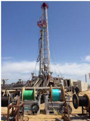
Figure 4.2-6. WIRE cable being installed at a well in Diatomite/Tulare Formation.
