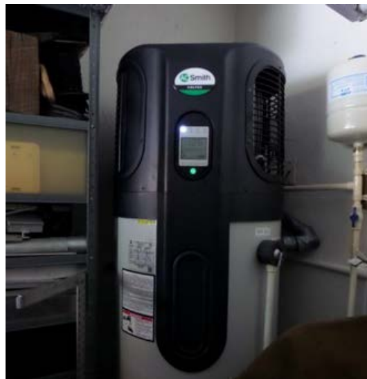
Figure 150. HPWH retrofit existing conditions
