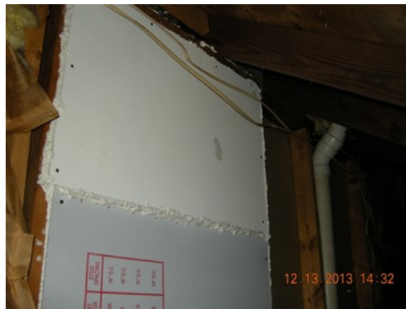
Figure 145. Air barrier installed
