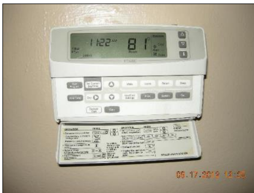
Figure 38: Site 28 existing thermostat, a Trane XT500C programmable model
