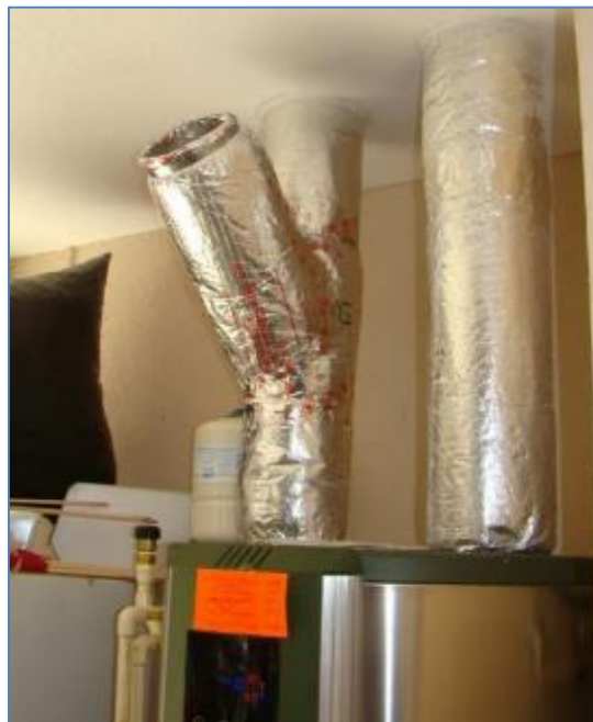
Figure 12. Y-type ducting arrangement at Site 5 allowing cold exhaust air to be diverted from the conditioned living environment
