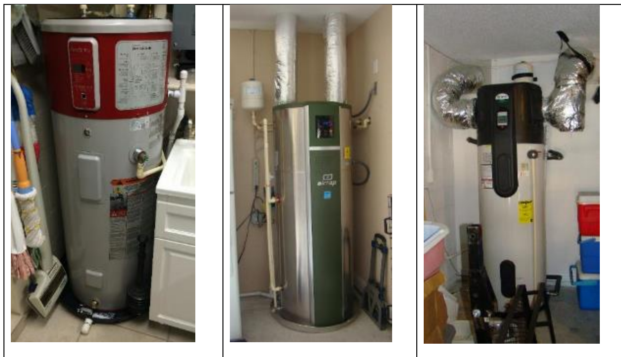
Figure 5. Heat pump water heater configurations: Left, interior GE unit in utility room at Site 13; center, ducted AirGenerate unit at Site 5; right, ducted A.O. Smith unit at Site 26
