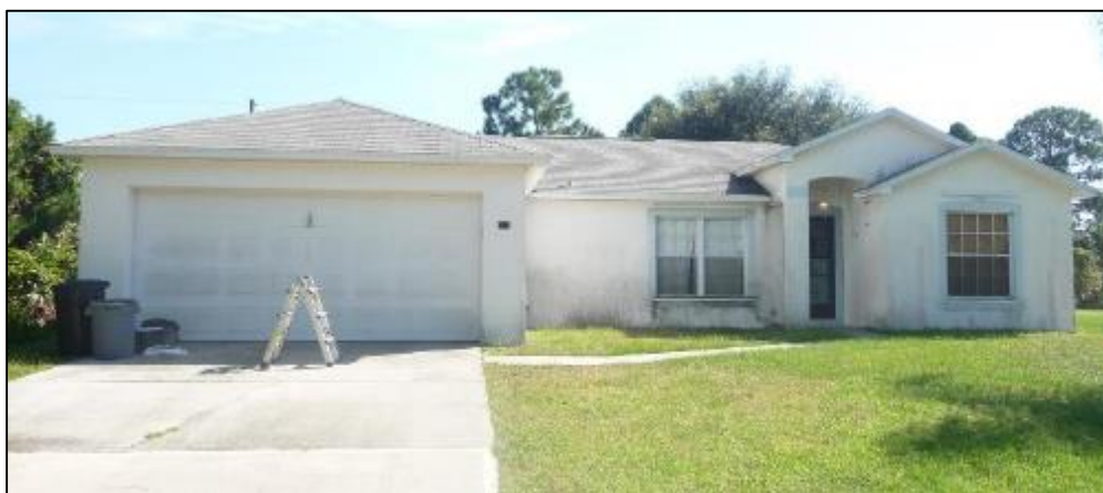
Figure 13. Site 54 Prior to EIFS and window retrofit
