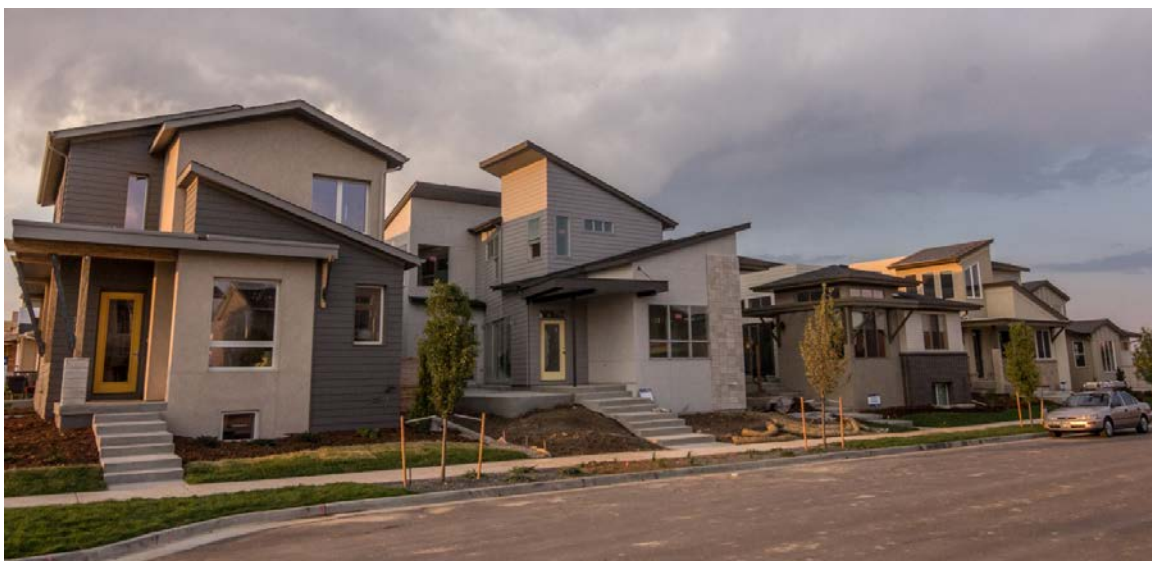
Figure 16. Test house (Passive House) (far left) and other production houses in Midtown
