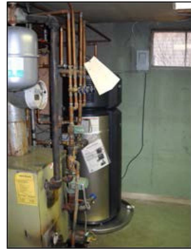
Figure 9. This HPWH benefited from the waste heat of the boiler used for space heating.
