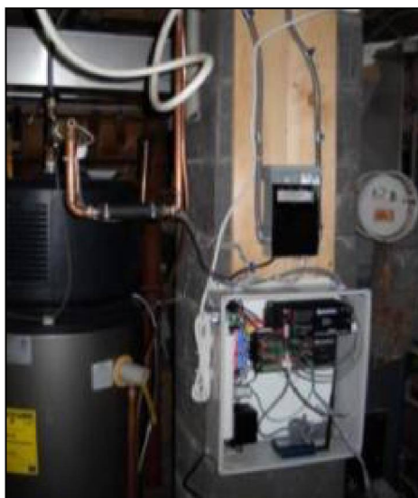
Figure 3. Example of an HPWH monitoring system installation
