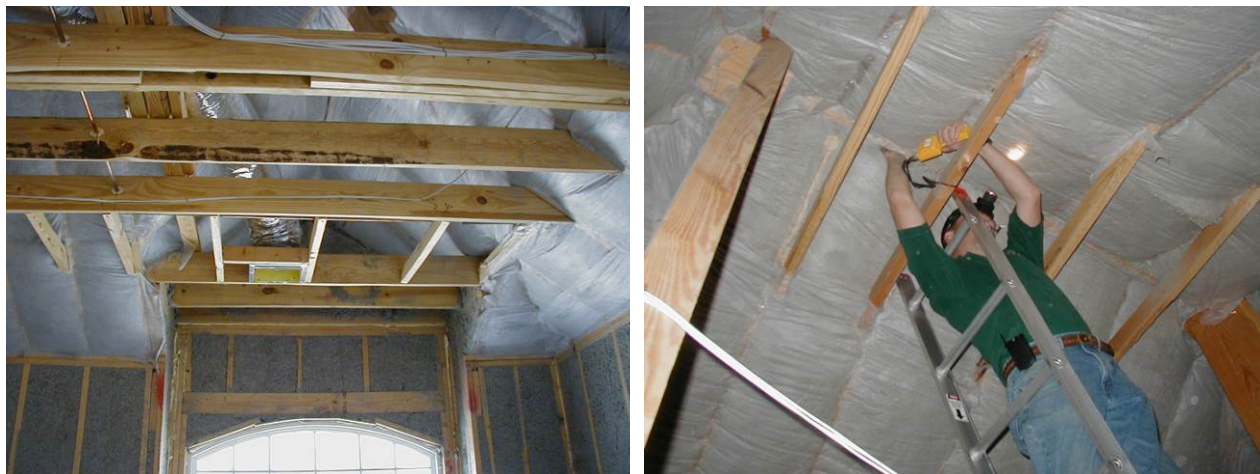
Figure 9. Netted and blown cellulose roof insulation in Houston (left); MC at the roof ridge (right)
