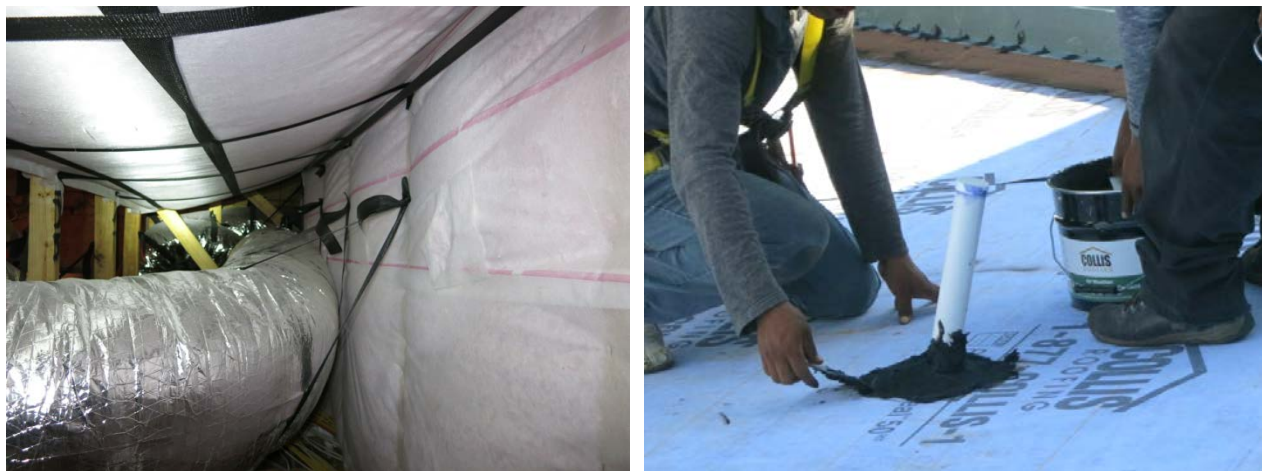
Figure 20. Insulated attic knee wall (left) and waterproofing/air barrier at roof penetration (right)
