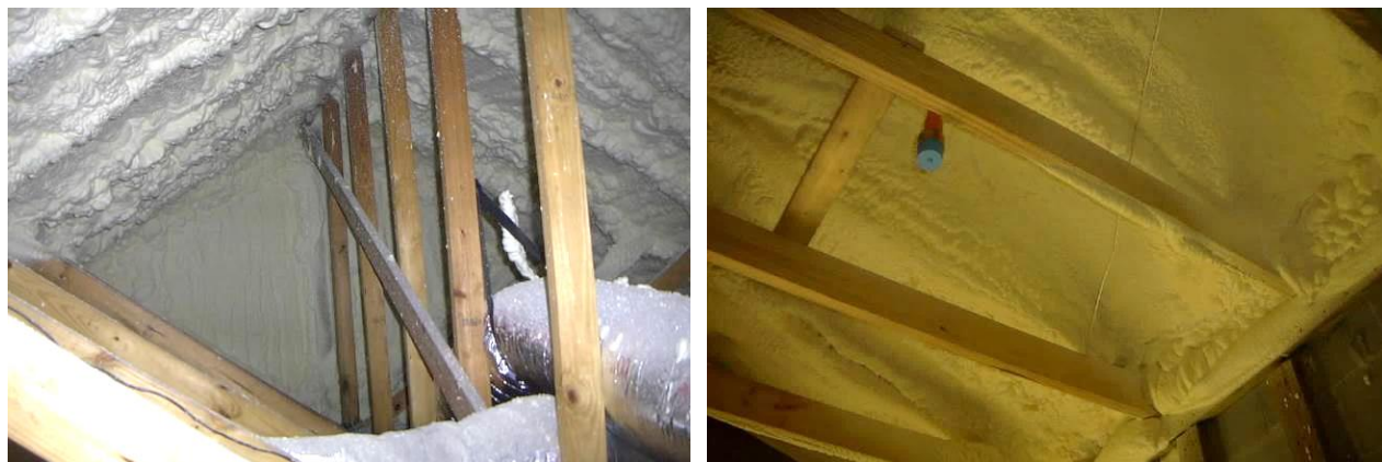
Figure 1. SPF unvented roofs
