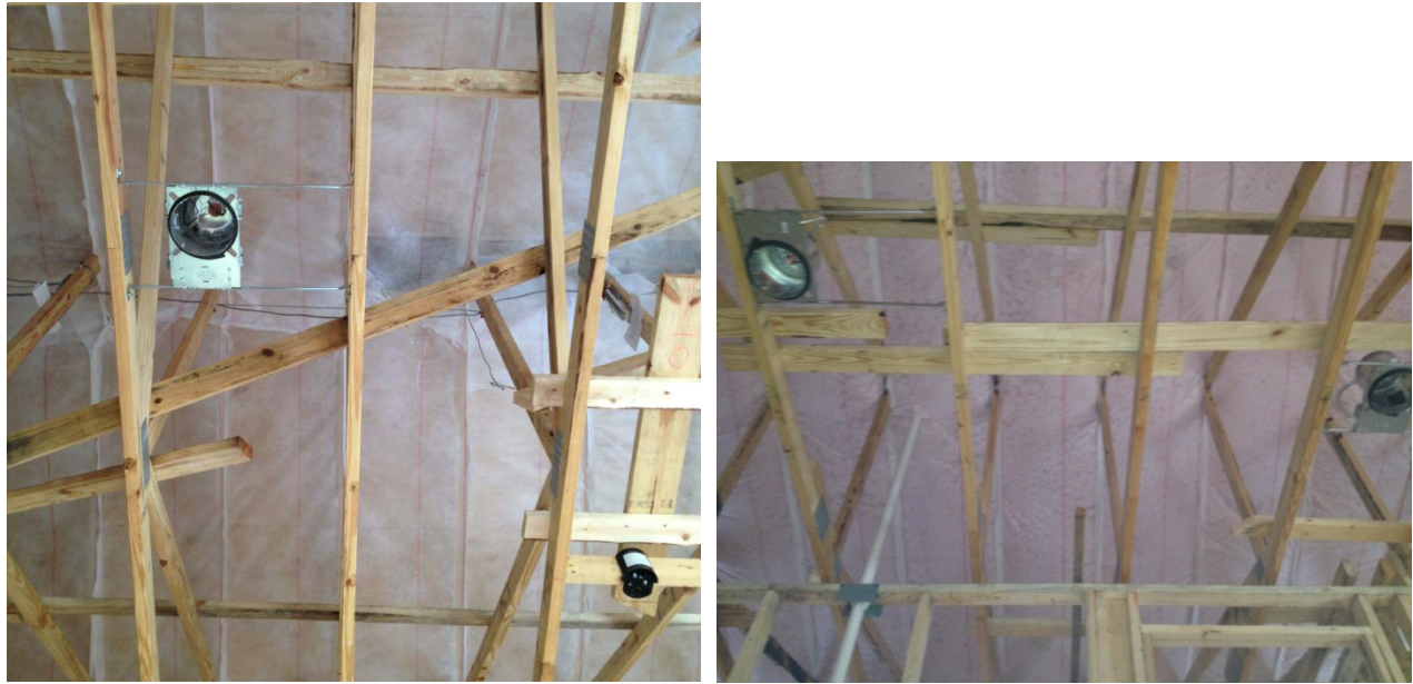
Figure 17. Boxed netting insulation system before (left) and after (right) insulation blowing
