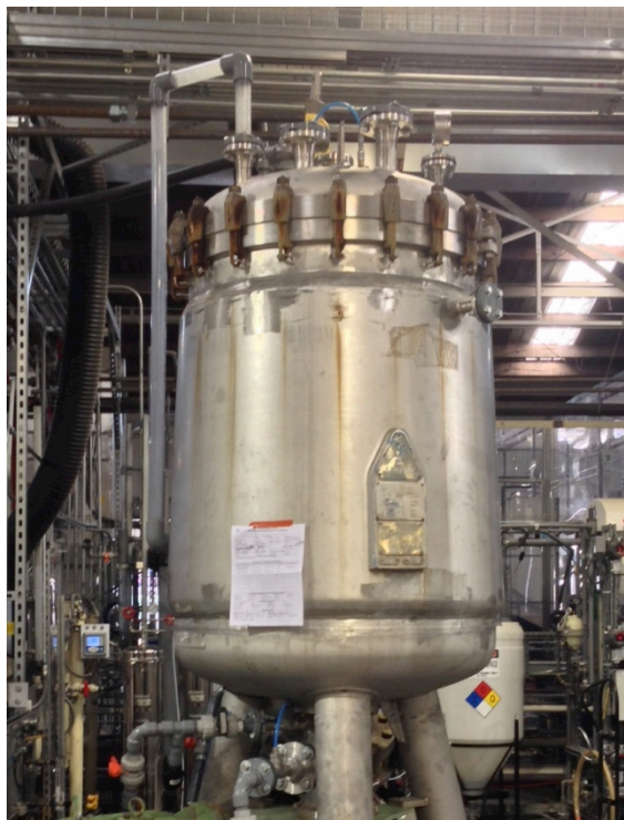
Figure 2-8 Centrifugal discharge filter used to remove impurities from dissolved waste oxide
