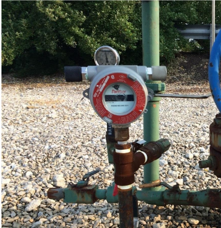
Figure 4-2. Pressure/Temperature Recording Gauge
