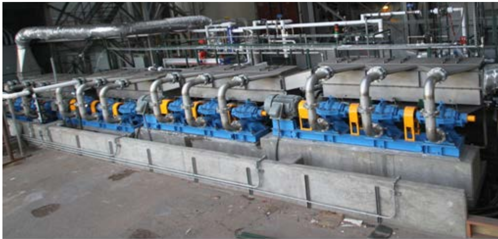
Figure 9: CARE NeuStream® CO 2 absorbers installed at the Drake plant
