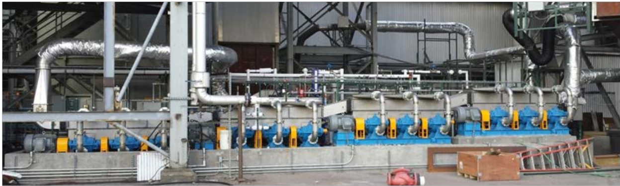
Figure 7: CARE system enclosure with containment berm at CSU's Martin Drake power plant
