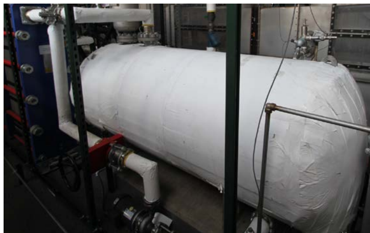
Figure 10: CARE stripper unit installed at the Drake plant
