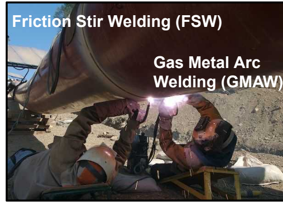
Welding to join or repair pipe
