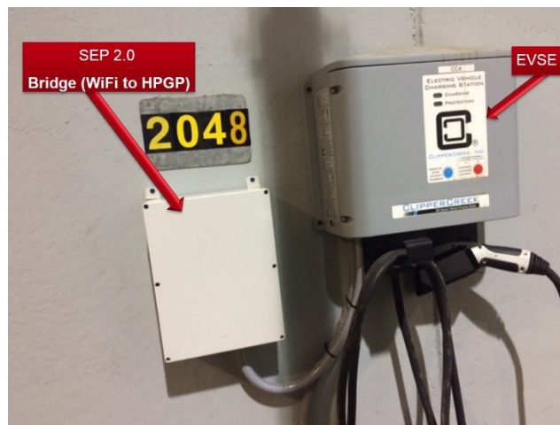
Figure 5-16 Communication box connected to electric vehicle supply equipment
