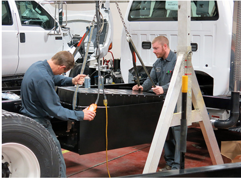
Figure 3-21 Installing a battery onto a chassis
