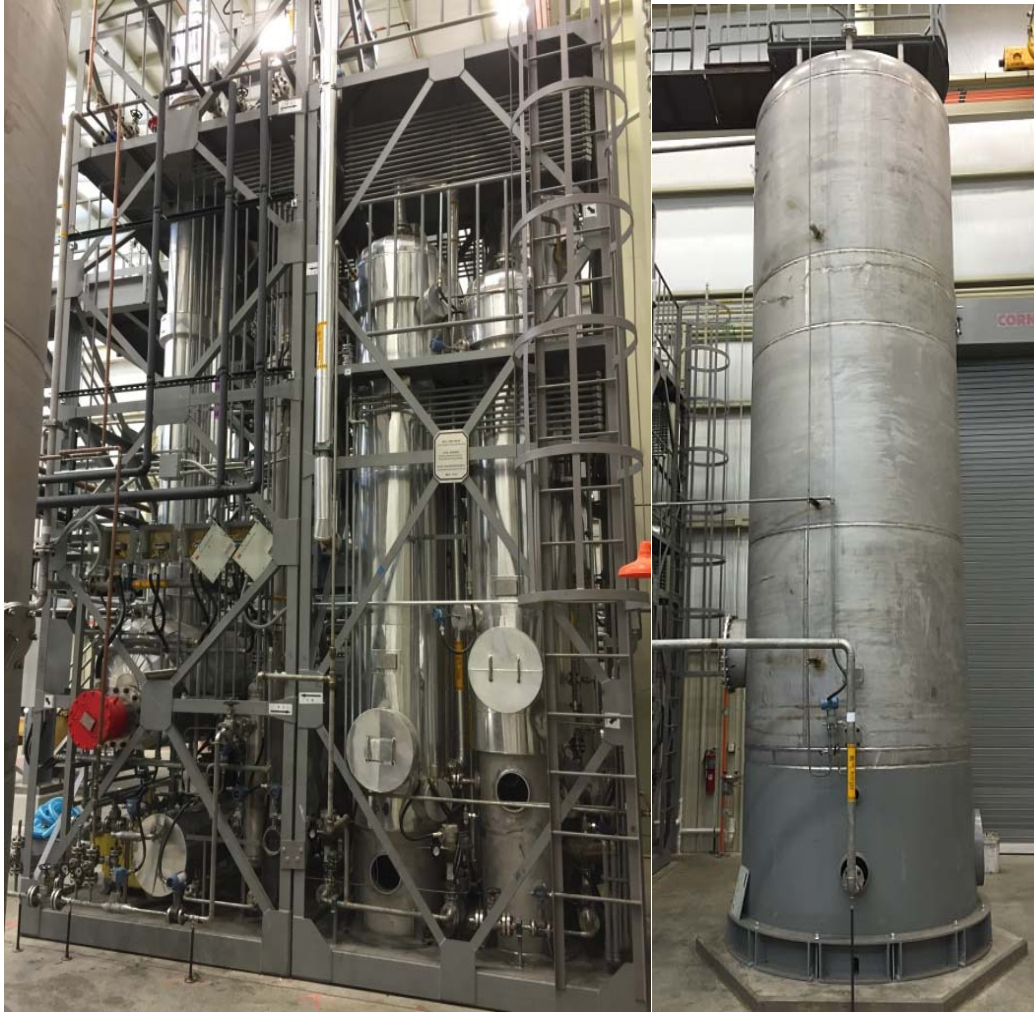
Figure 15: Photo - Acid Gas Removal Unit (left) and Activated Carbon Bed (right)
