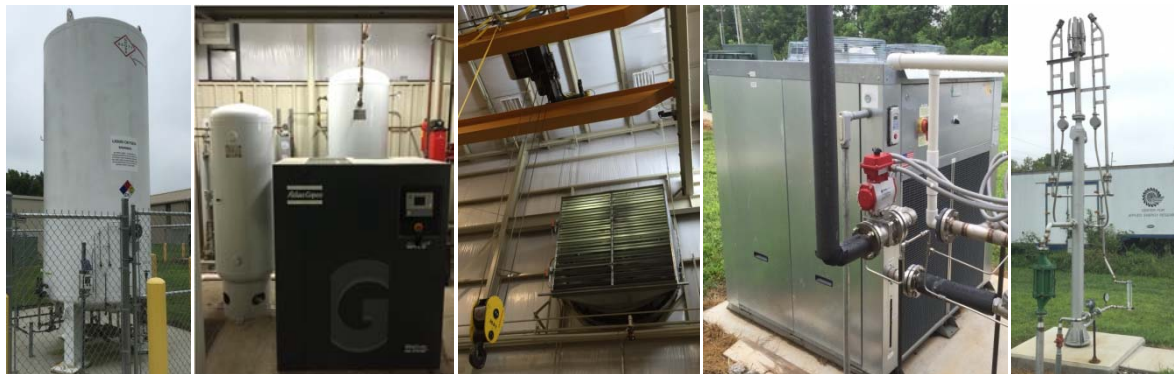
Figure 17: Photo – O2 Tank, Compressor, N2 Generator, Crane, Safety Fans, Chiller, Flare.
