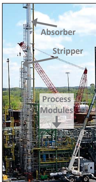
Figure 89. Installation of the Linde-BASF Pilot Unit
