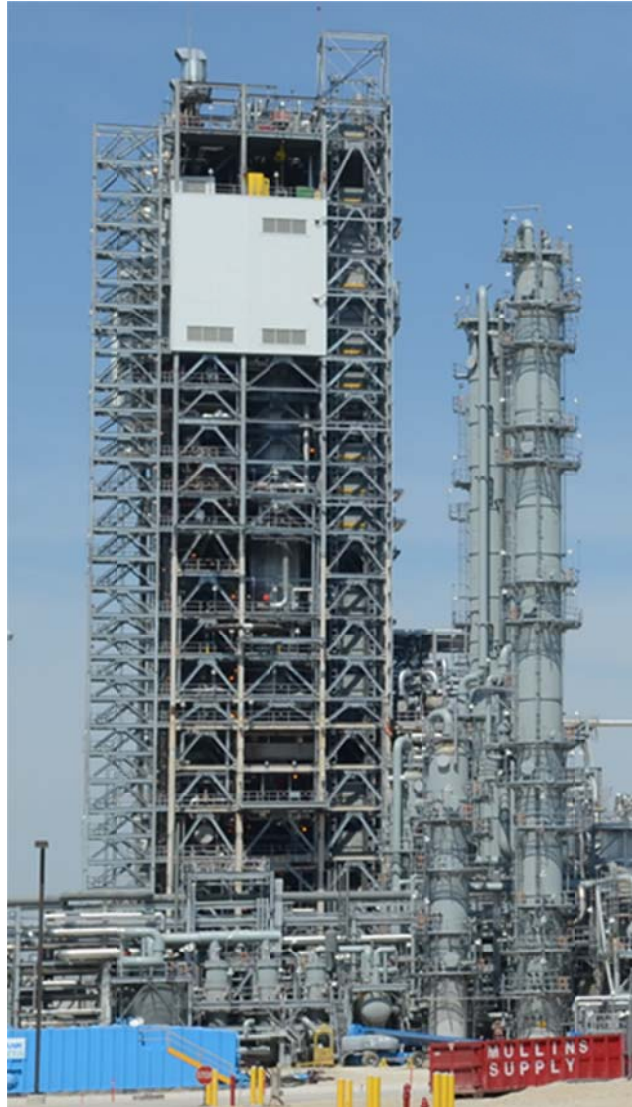
Figure 2.4: Edwardsport, IN; IGCC Photo of Gasifier Island Structure From Duke Energy, Edwardsport, IN IGCC website http://www.duke-energy.com/about-us/edwardsport-overview.asp
