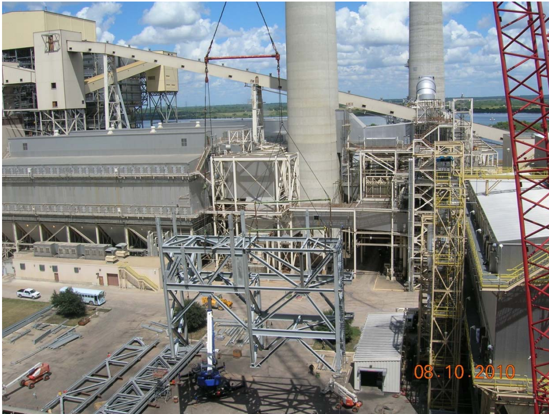
Figure A.3: Example of Kiewit project using modularization for a pipe rack type structure.
