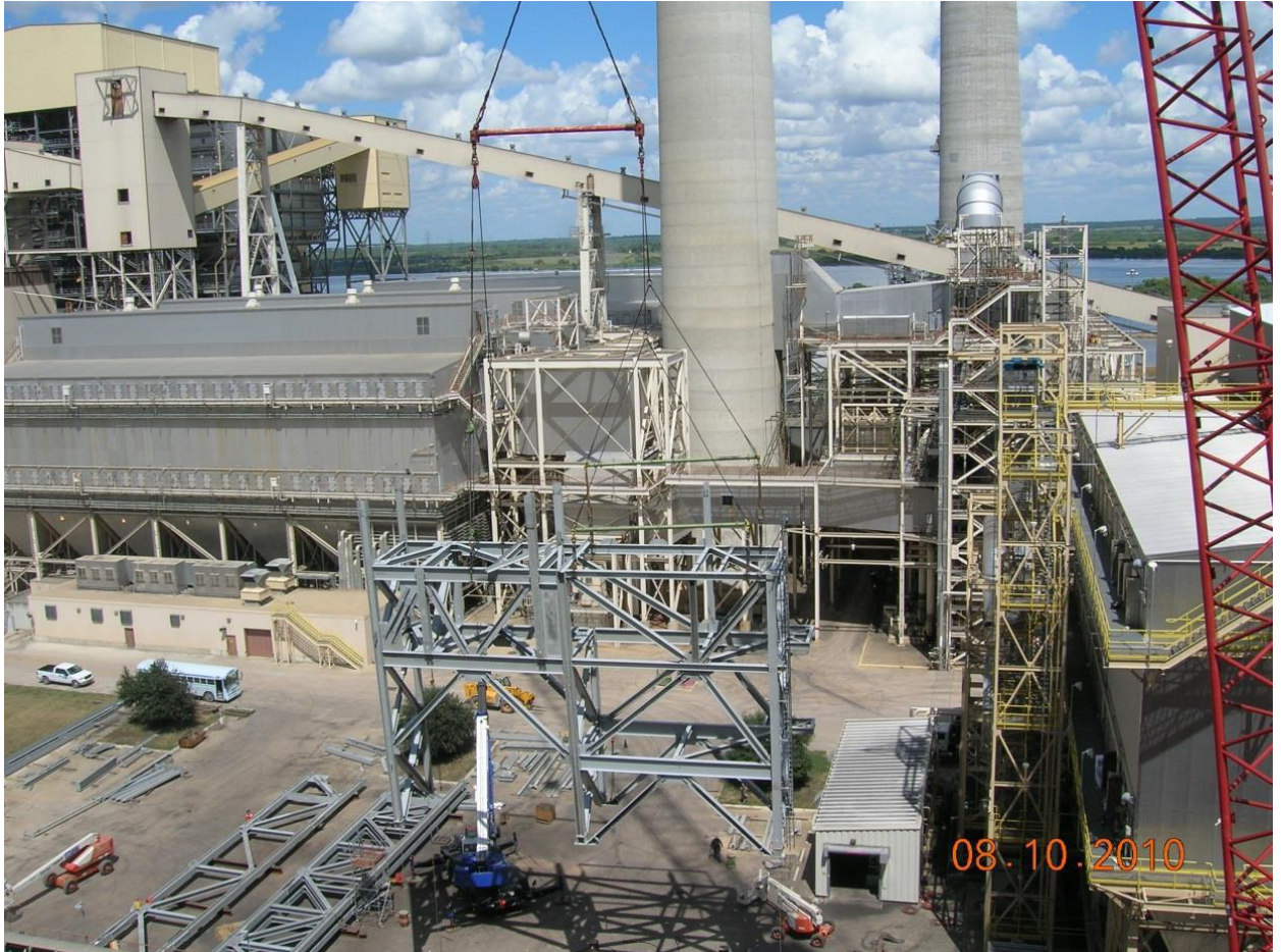
Figure 3. Example of Kiewit project using modularization for a pipe rack type structure
