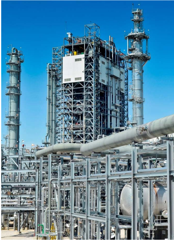
Figure A.2: Example of Pipe Rack with Gasifier Island in Background http://www.duke-energy.com/about-us/edwardsport-overview.asp
