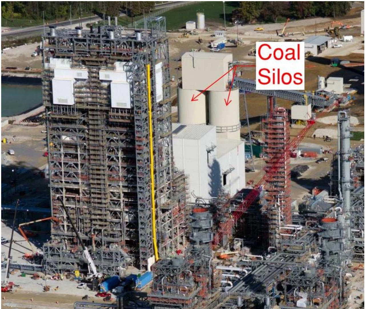
Figure A.1: Silo Storage Structures are excellent candidates for the Concrete Slip Form Method.
