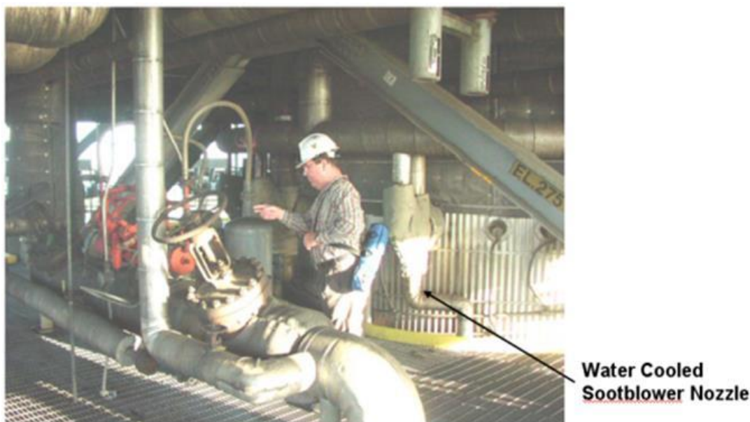
Figure 13. Soot blowers at TECO (Tampa Electric Company 2002).
