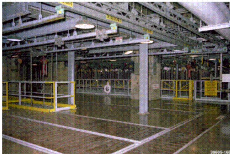
Figure 10. Storage Basin Monorail System
