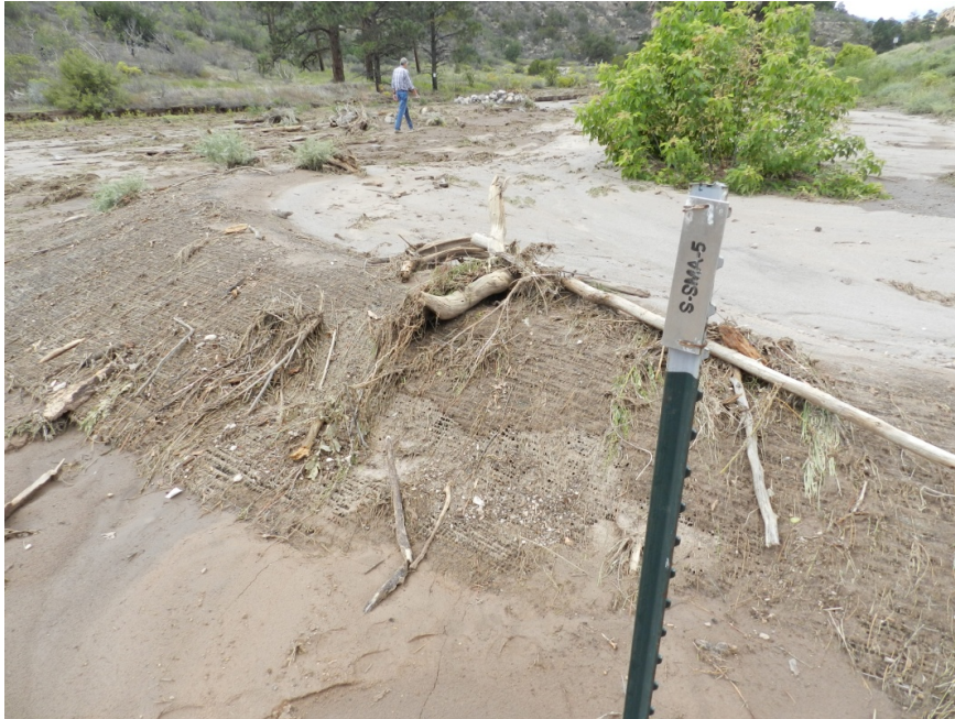
Figure 15 S-SMA-5 Control berm damaged and filled with sediment. ISCO automated sampler and battery found downstream.
