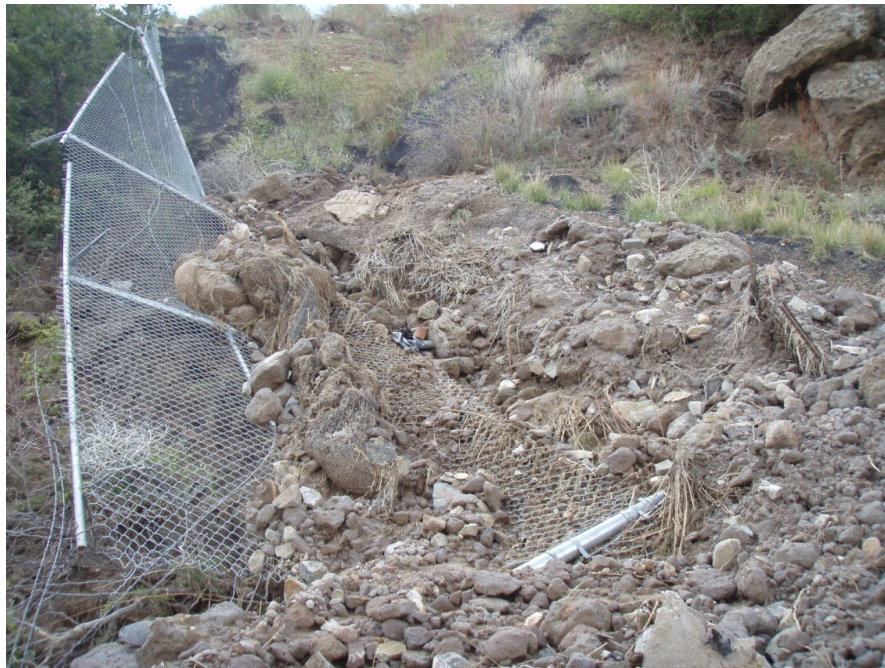
Figure 9 Slope failure at P-SMA-1
