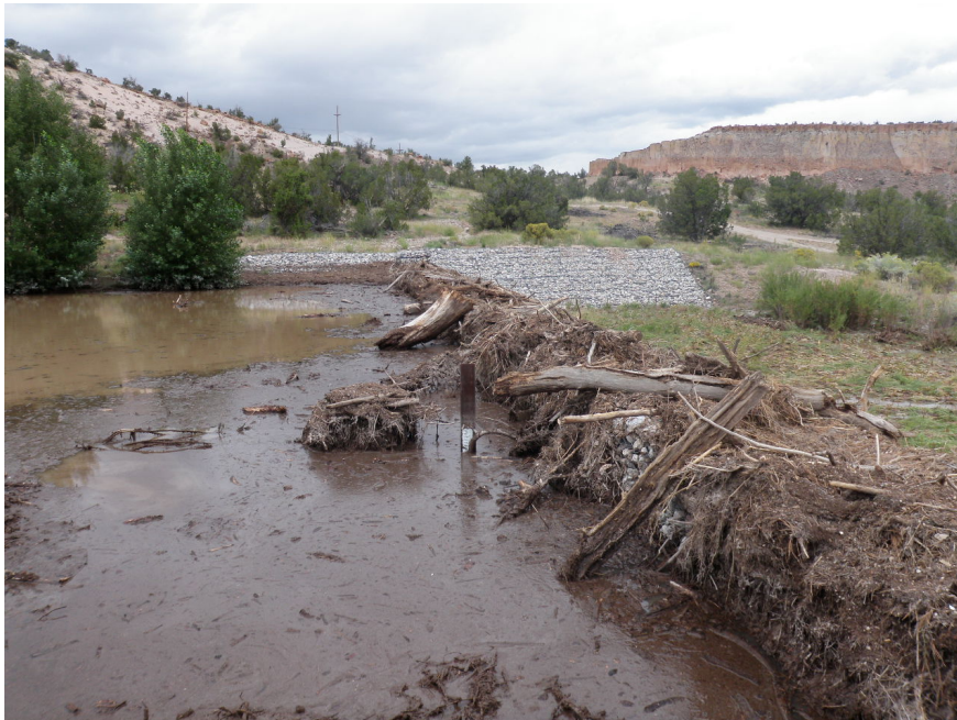
Figure 8 Flood debris at the Los Alamos Canyon weir spillway
