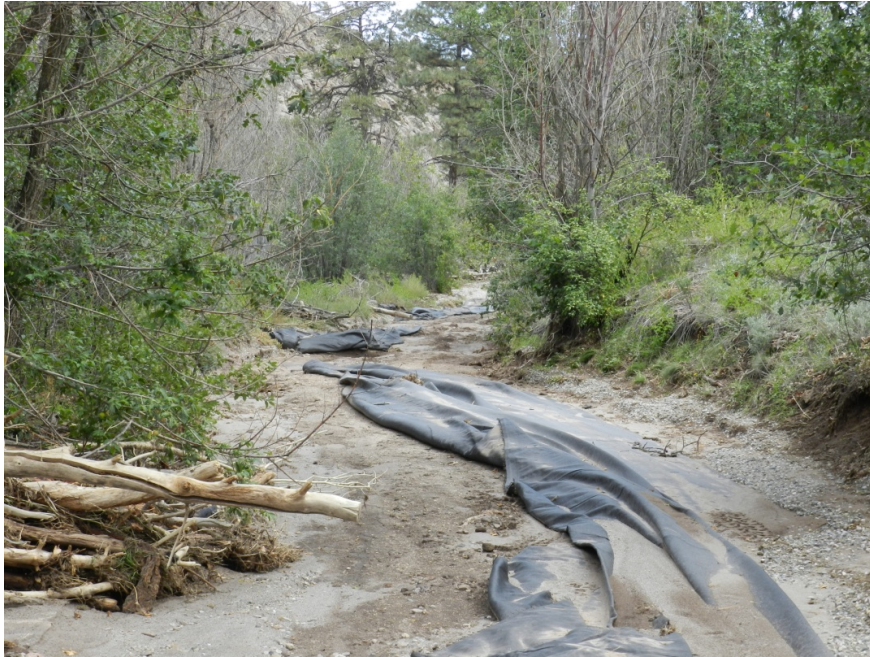
Figure 12 Damaged access road above sediment traps in Mortandad Canyon
