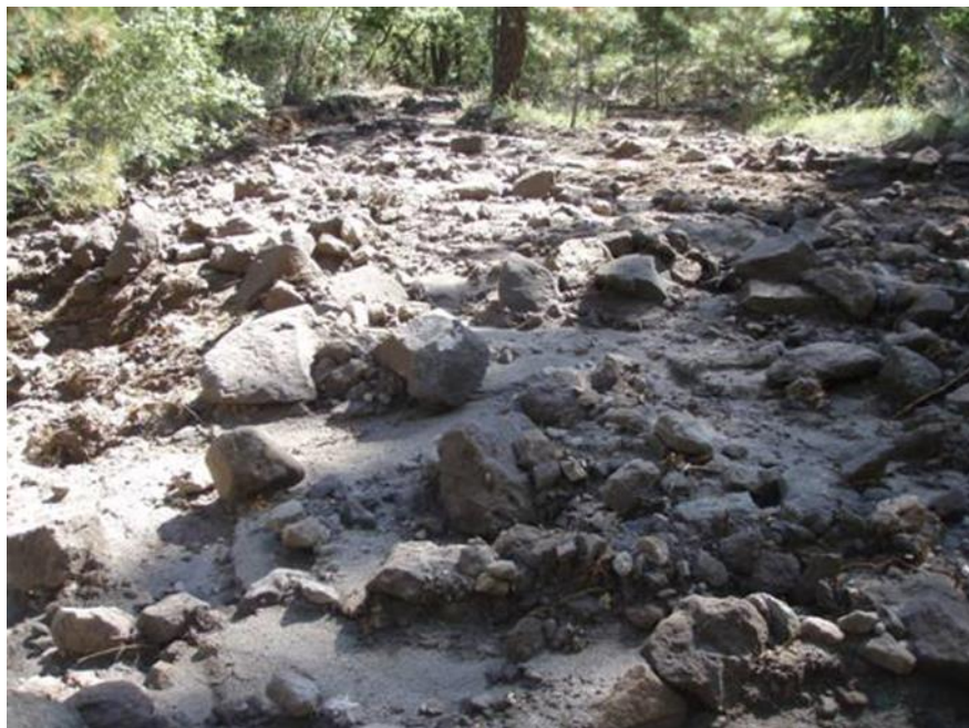
Figure 18 Damaged access road in Water Canyon
