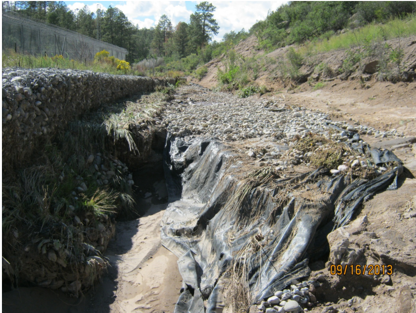
Figure 10 Damage to Threemile Canyon access road
