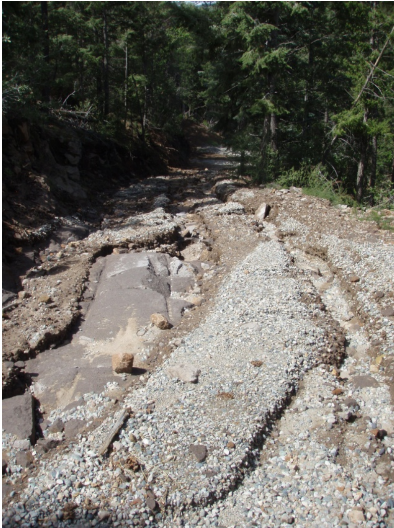
Figure 16 Damage to Cañon de Valle access road
