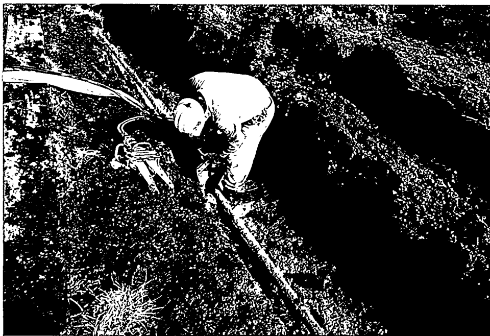
Figure 4.2 The Pneumatic Transfer Tube Was Crimped Before Being Cut (ANL Neg. 24692K, Frame 24)
