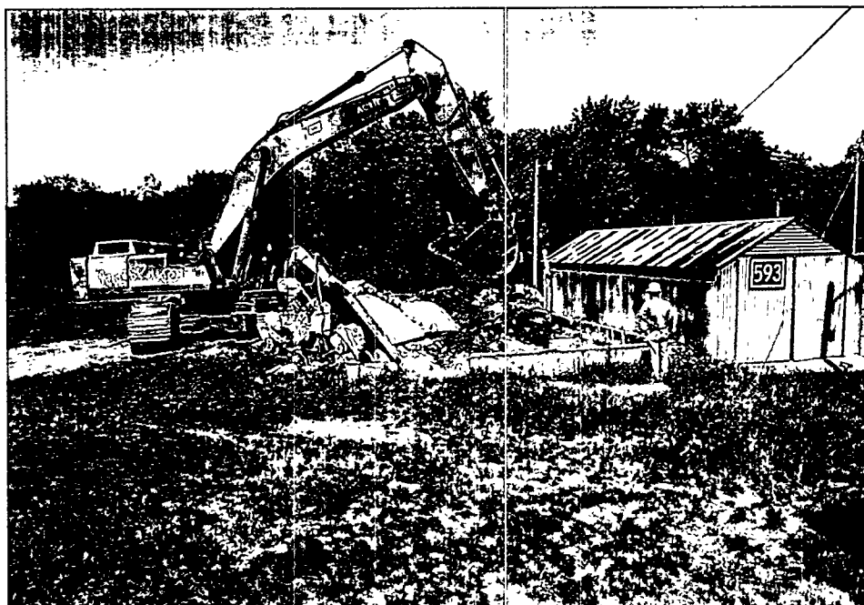
Figure 6.4 Removal of Concrete Pad (ANL Neg. # 24693, Frame 2)
