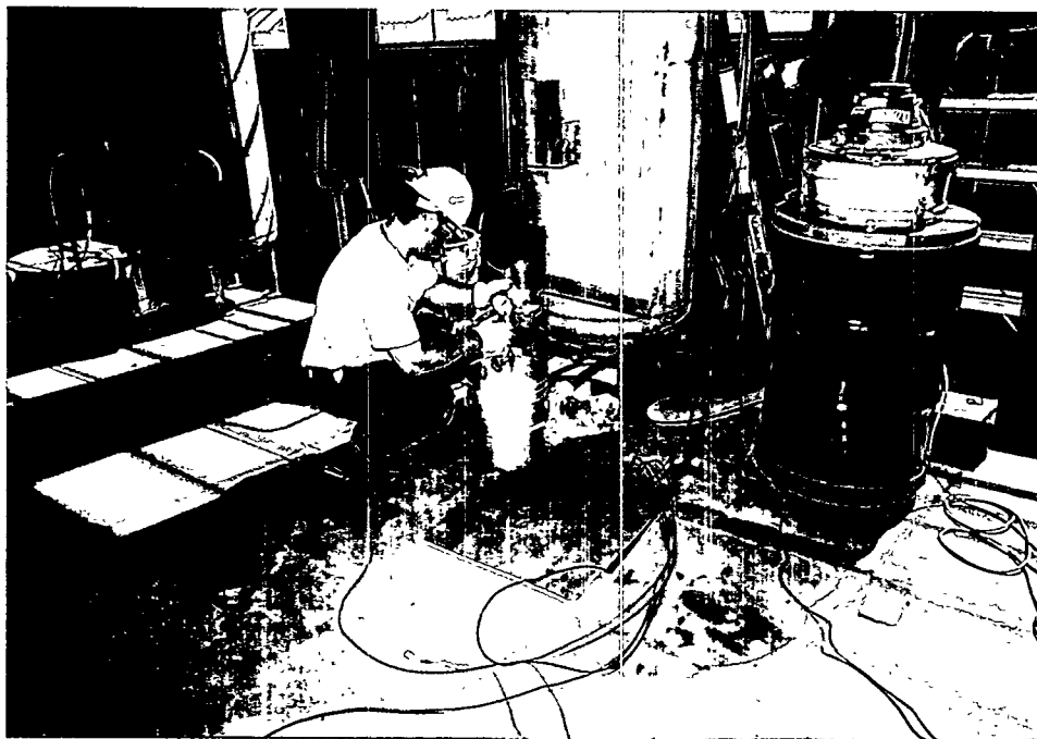
Figure 6.1 WMO Technician Draining a Waste Ion Exchange Tank (ANL Neg. # 24344K, Frame 11)
