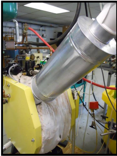
Figure 18: Heat exchanger installation
