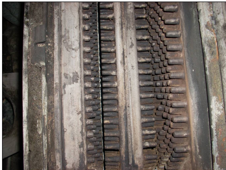
Boiler Inside Flue Passage After Cleaning
