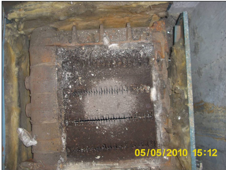
Boiler Inside Flue Passage Before Cleaning
