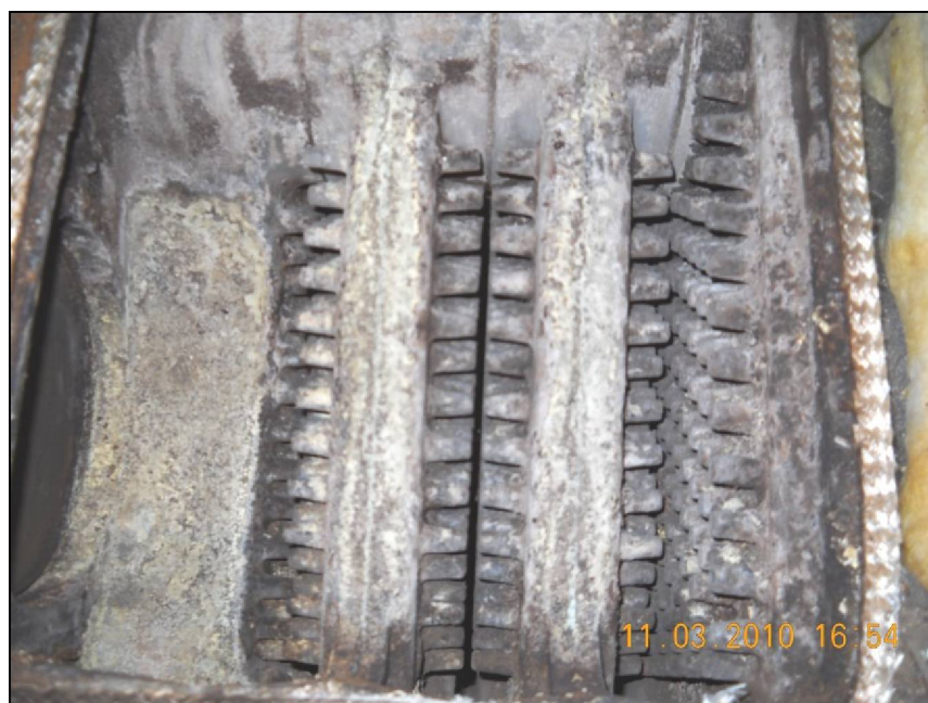
Boiler Inside Flue Passage After Cleaning
