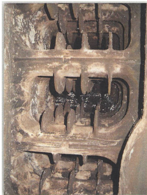
Boiler Inside Flue Passage After Cleaning
