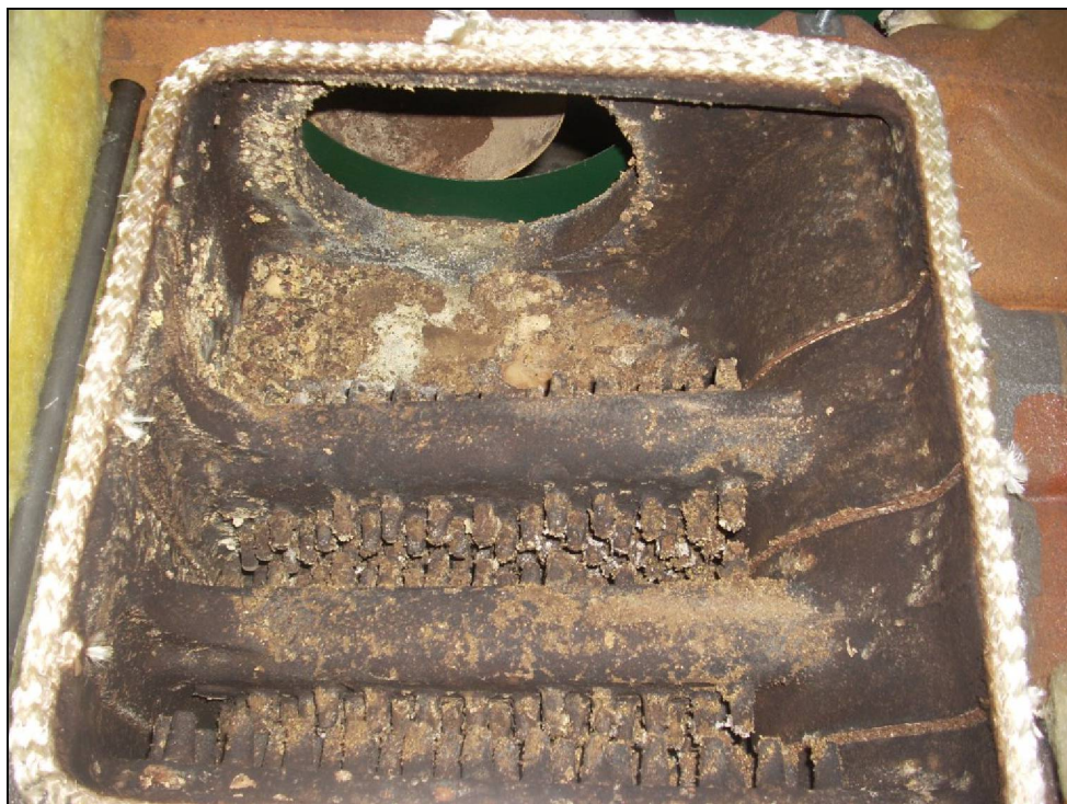
Boiler Inside Flue Passage Before Cleaning
