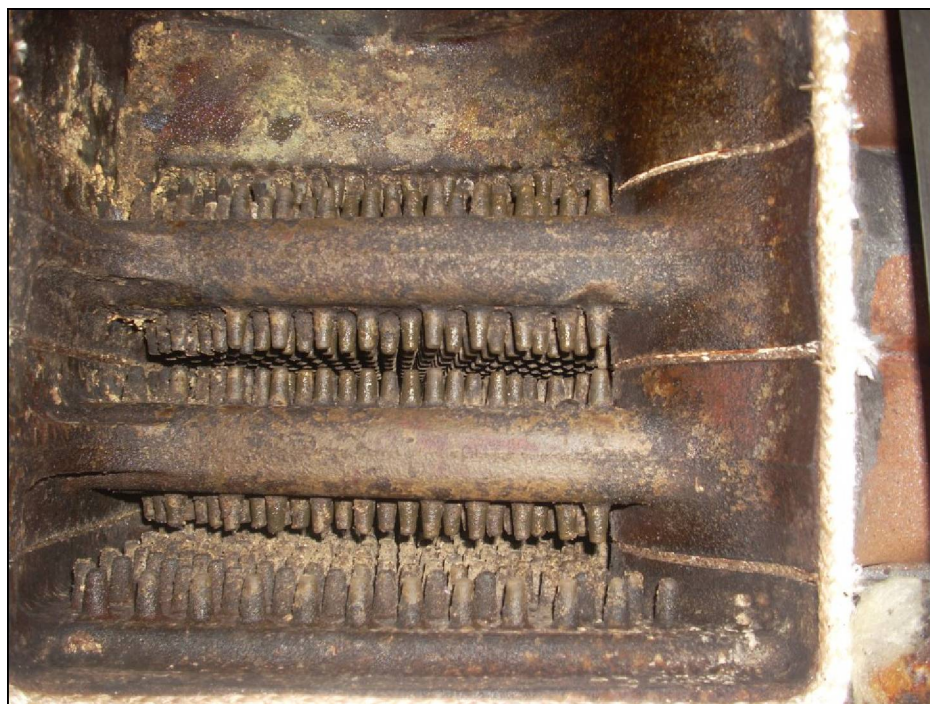
Boiler Inside Flue Passage After Cleaning
