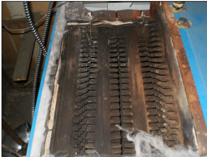
Boiler Inside Flue Passage After Cleaning
