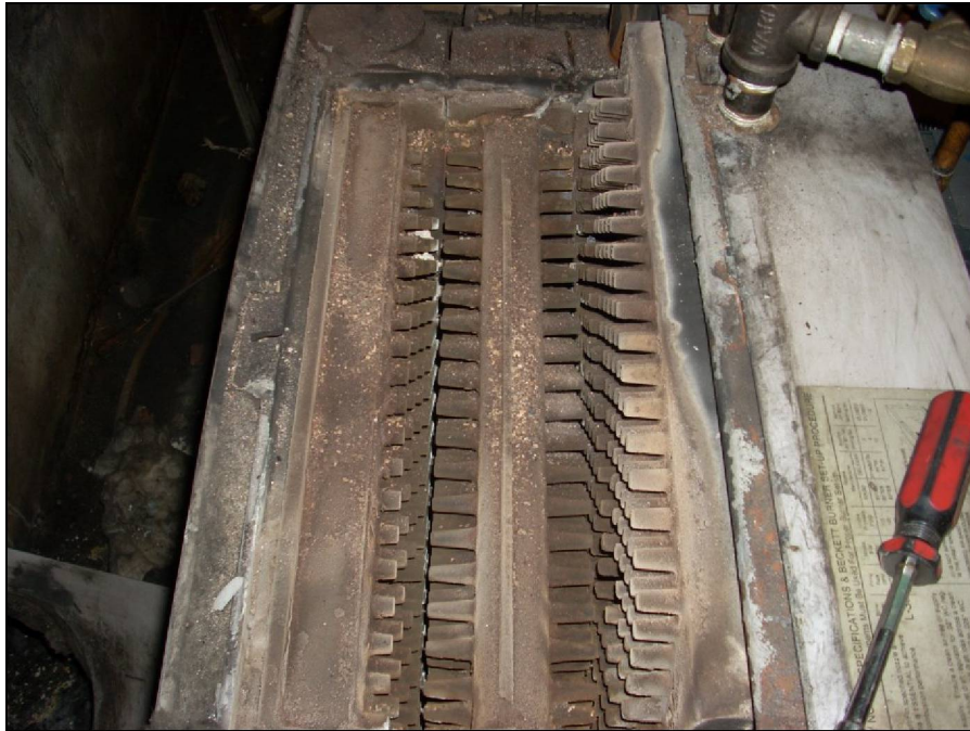
Boiler Inside Flue Passage Before Cleaning
