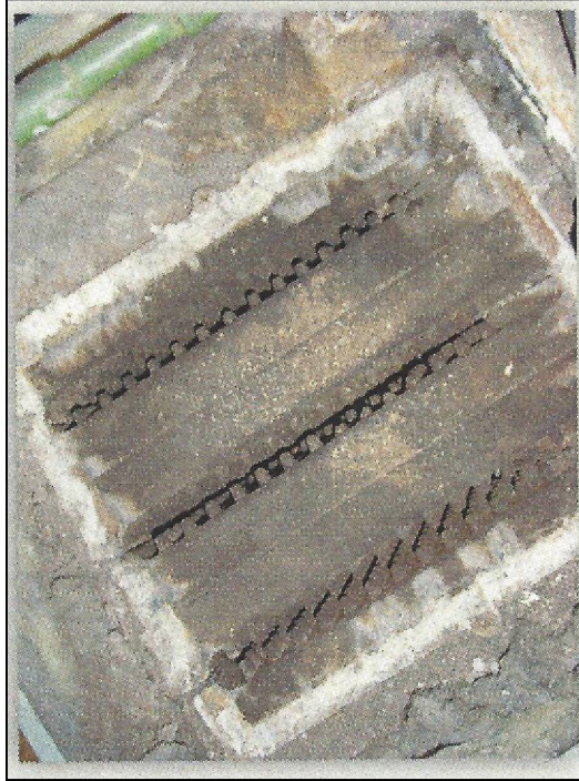
Boiler Inside Flue Passage Before Cleaning
