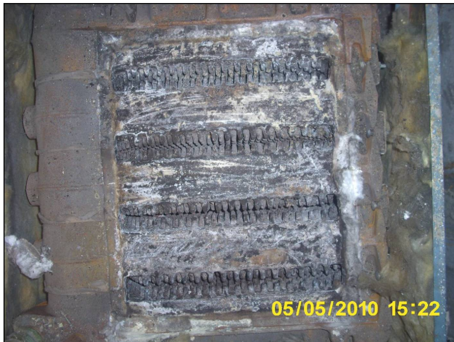
Boiler Inside Flue Passage After Cleaning
