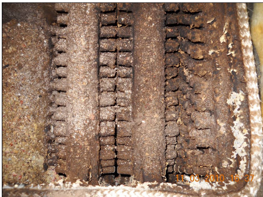
Boiler Inside Flue Passage Before Cleaning
