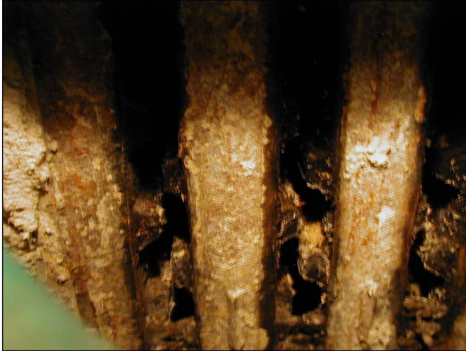
Boiler Inside Flue Passage Before Cleaning
