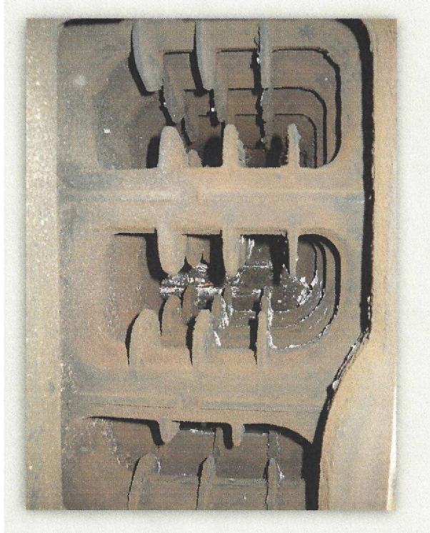
Boiler Inside Flue Passage Before Cleaning
