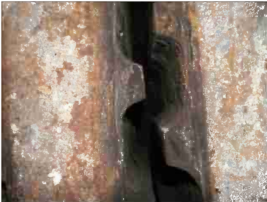
Boiler Inside Flue Passage After Cleaning
