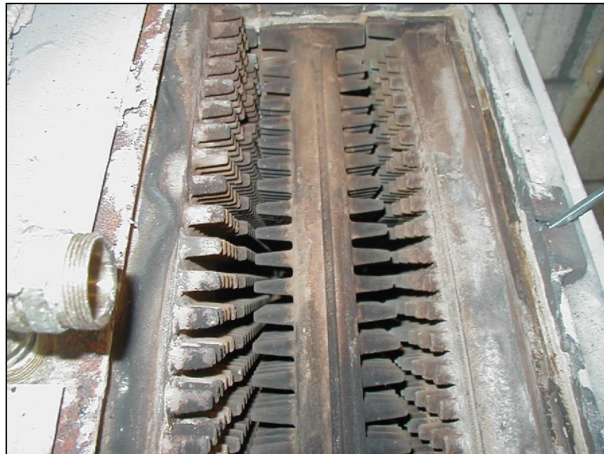
Boiler Inside Flue Passage After Cleaning
