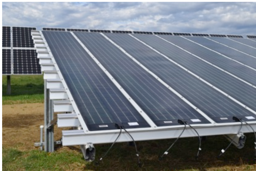
Figure 31. Global Solar CIGS modules at the Vermont RTC that are being installed by PVMC.
