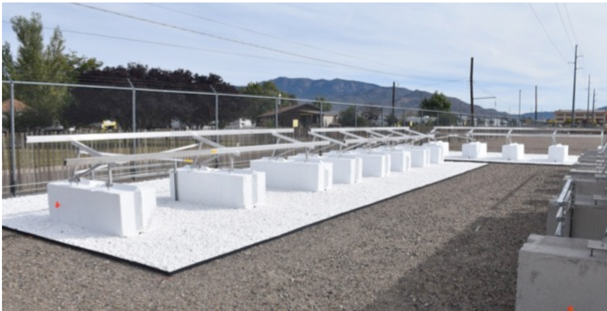
Figure 28. Portion of the Prism installation in New Mexico. Some of the racks are placed on a highly reflective white background to enhance the light available on the back of the arrays.
