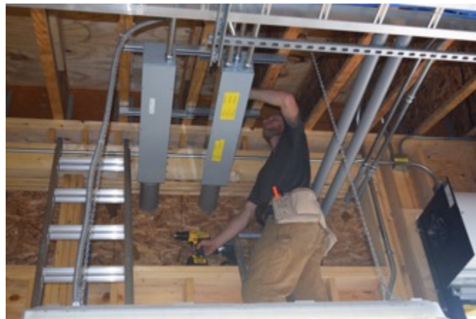
Figure 34. Norwich Technologies reinforces the rafters in preparation for the EZ-PV installation.
