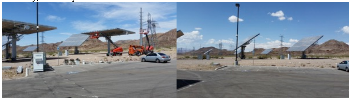
Figure 7. Left: Two Amonix trackers in foreground before removal. Right: site after all three trackers were removed and the site graded.
