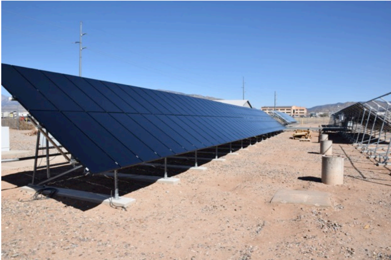
Figure 24. Stion system in New Mexico. Framed subarray in the foreground and frameless in the background.
