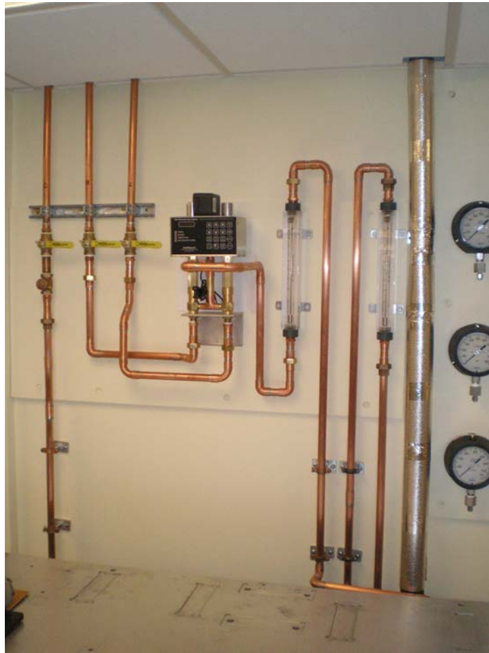
Figure 5-6: Cooling Water Supply, Flow Control, and Drain Plumbing Arrangement
