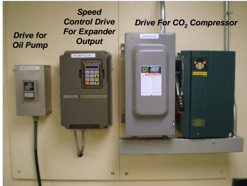
Figure 5-2: VFDs for CO 2 Expander Testing
