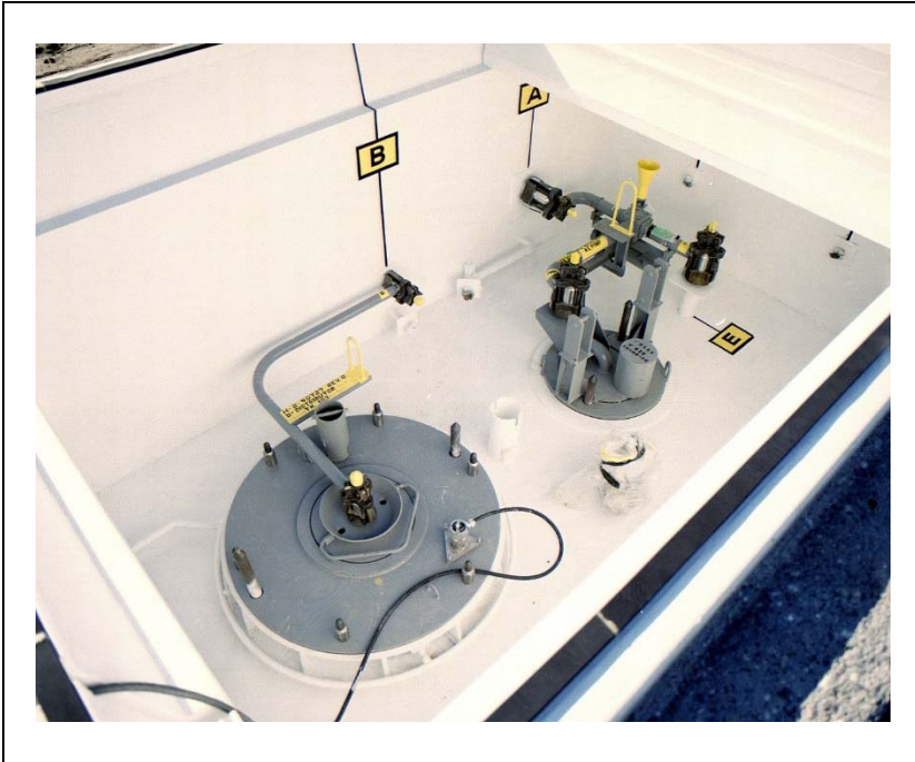
Fig. 2. Tank Farm Pump Pit with Concrete Shielding Cover Blocks Removed to Illustrate Typical Pipe Jumper Installation
