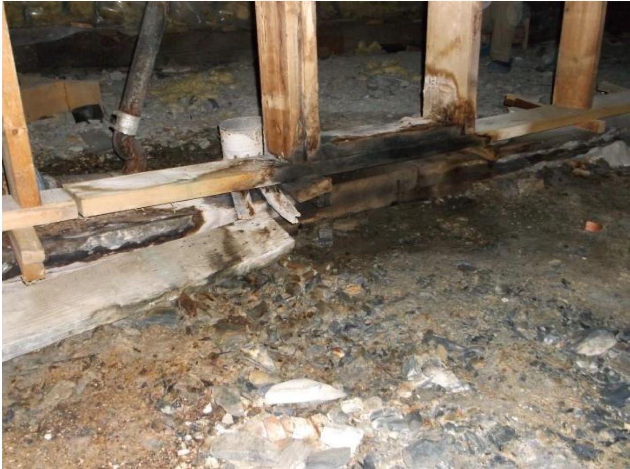
Figure 3. Mold and rot visible throughout the building's crawl space from various leaks and moisture issues. The building's knee walls were failing in some points when work was started but the knee walls would be shored up and repaired over the course of the project
