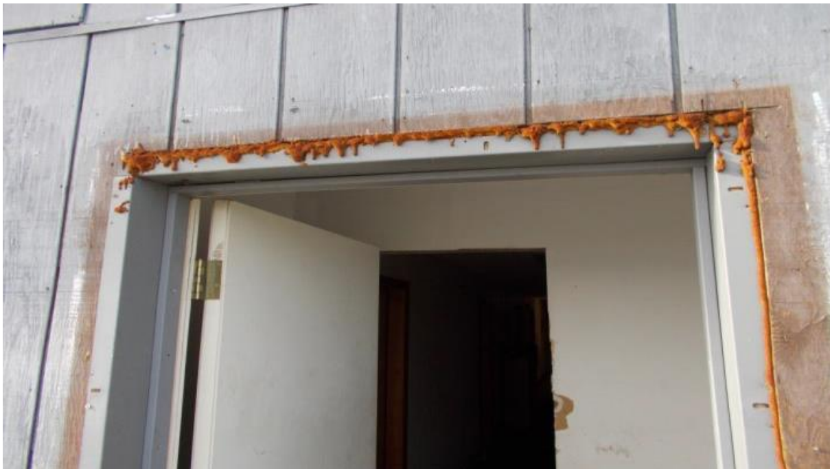
Figure 2. This was one of the older doors on the lodge, insulated around the frame but still with numerous air leaks around the entire frame and UV rays are reducing the effectiveness of the insulation
