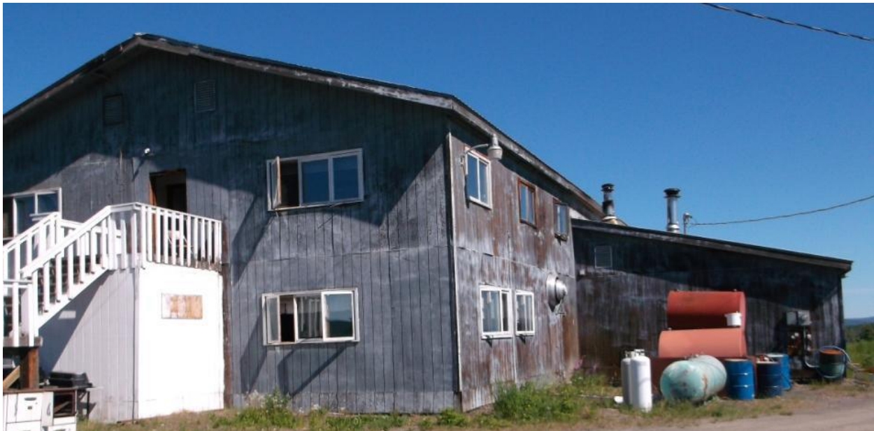
Figure 1 Old View of the Minto Lakeview Lodge from the same aspect as Figure 1 before Renovation. Note the stains on the building from 30+ years of frost buildup as the heat from inside the building met the extreme cold temperatures on the outside
