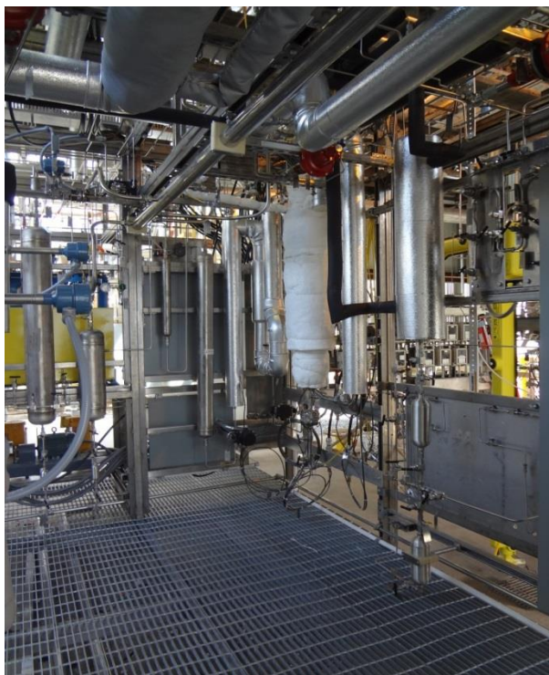
Figure 6. Guard beds, FT reactor and product collection
