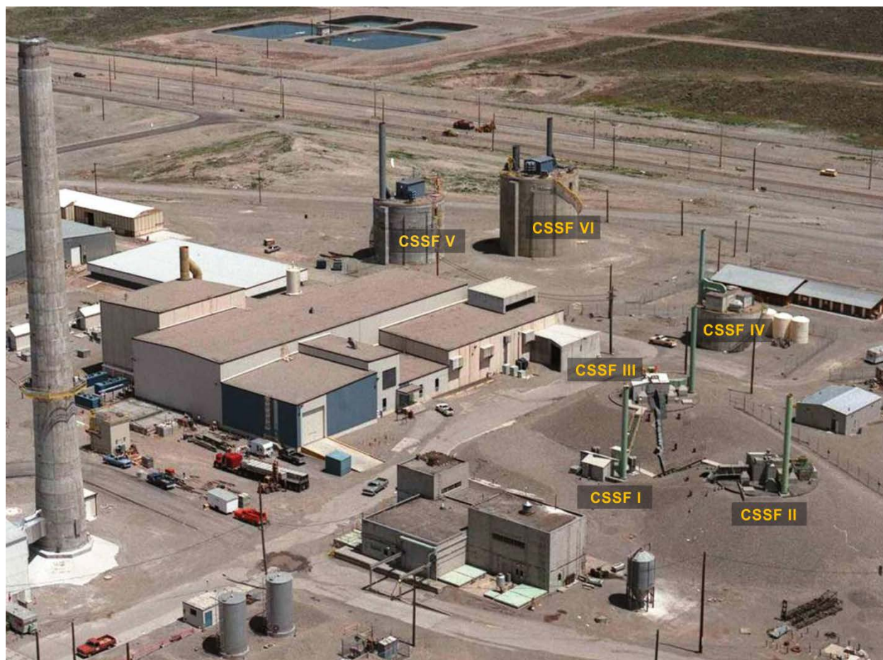
Figure 4-5. Photograph Showing the Locations of the Six CSSFs Containing Waste
