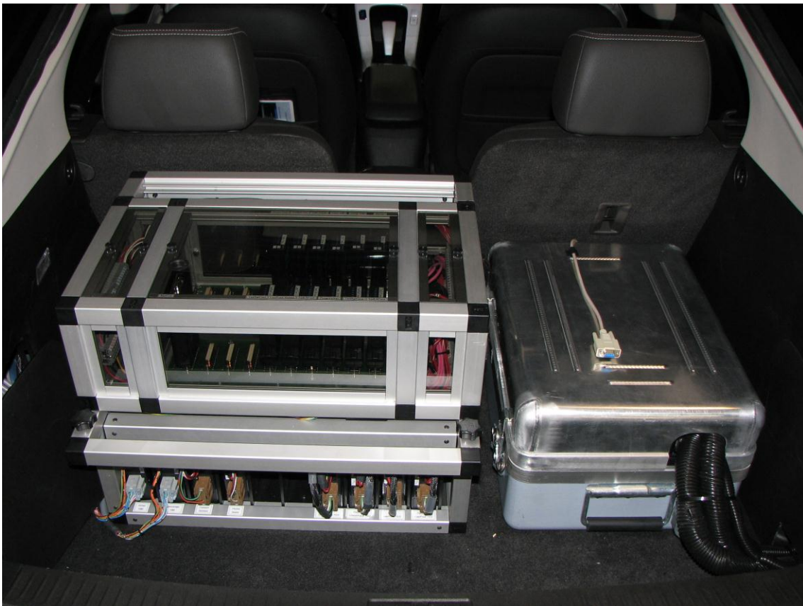
Figure G97: TE Controller Unit and CR9000X Data Logger Located in Volt Trunk
