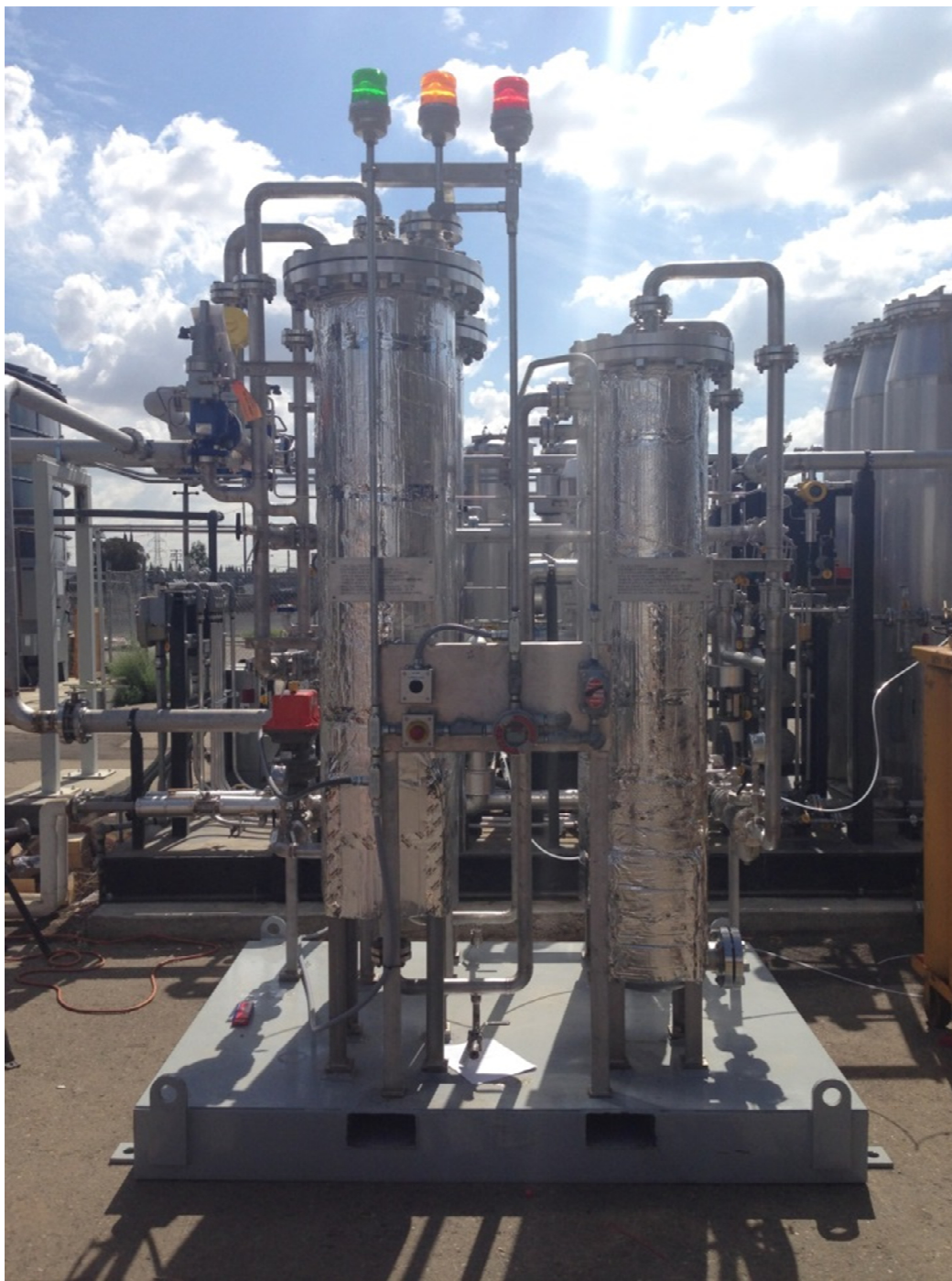
Figure 45. Picture of Sulfur Polishing Skid Installed at SATS.
