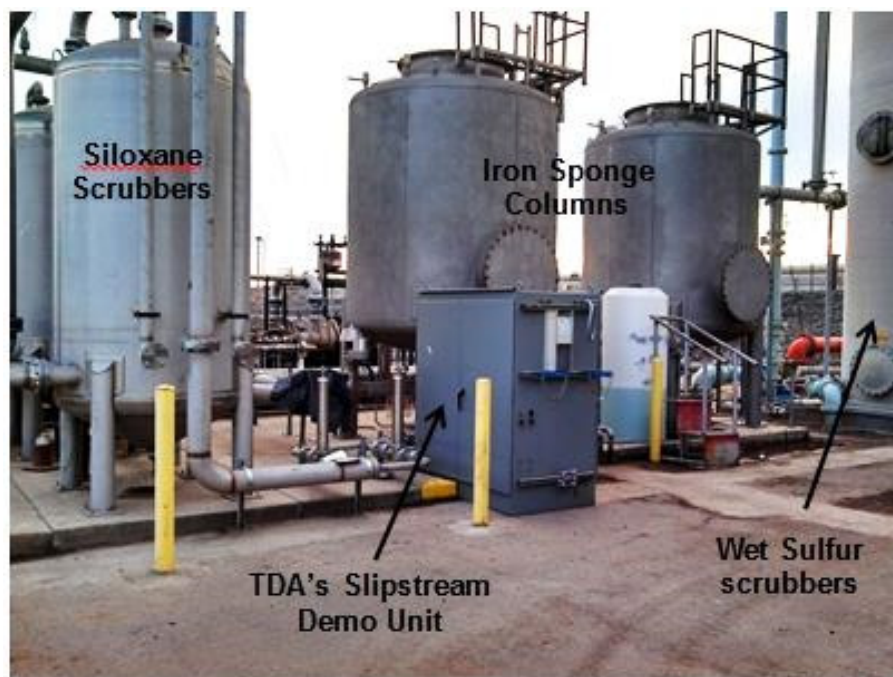
Figure 31. Test skid at Tulare Wastewater Treatment Plant.
