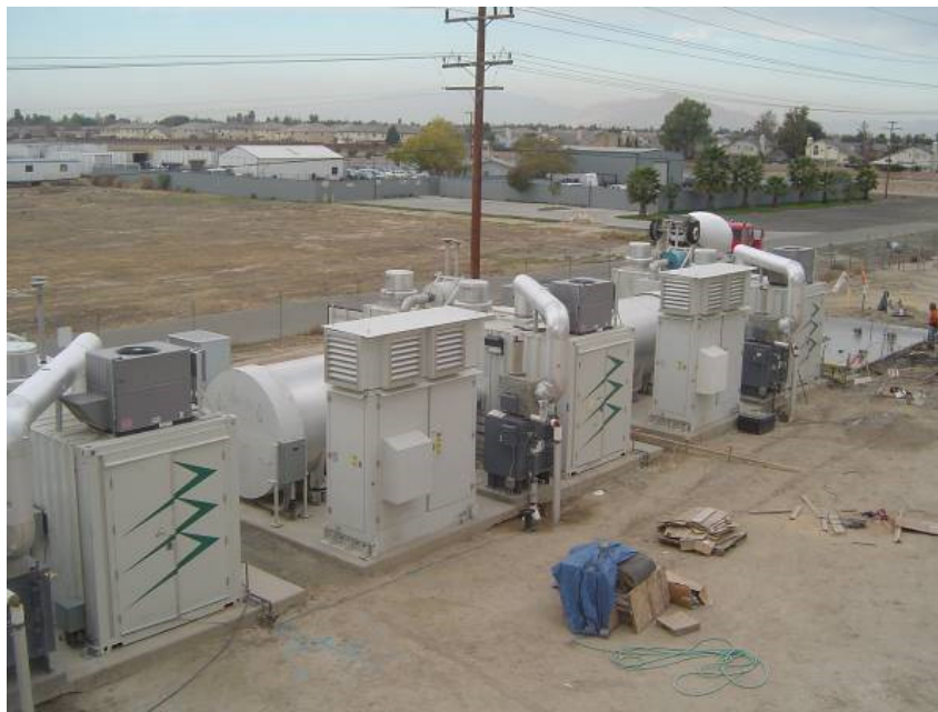
Figure 23. FCE's MCFC (DFC® units) installed at the Moreno Waste Water Treatment Facility (WWTF).
