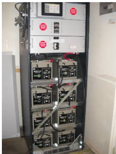
Figure 13.2: 9-kW SP Unit with Cover Removed
