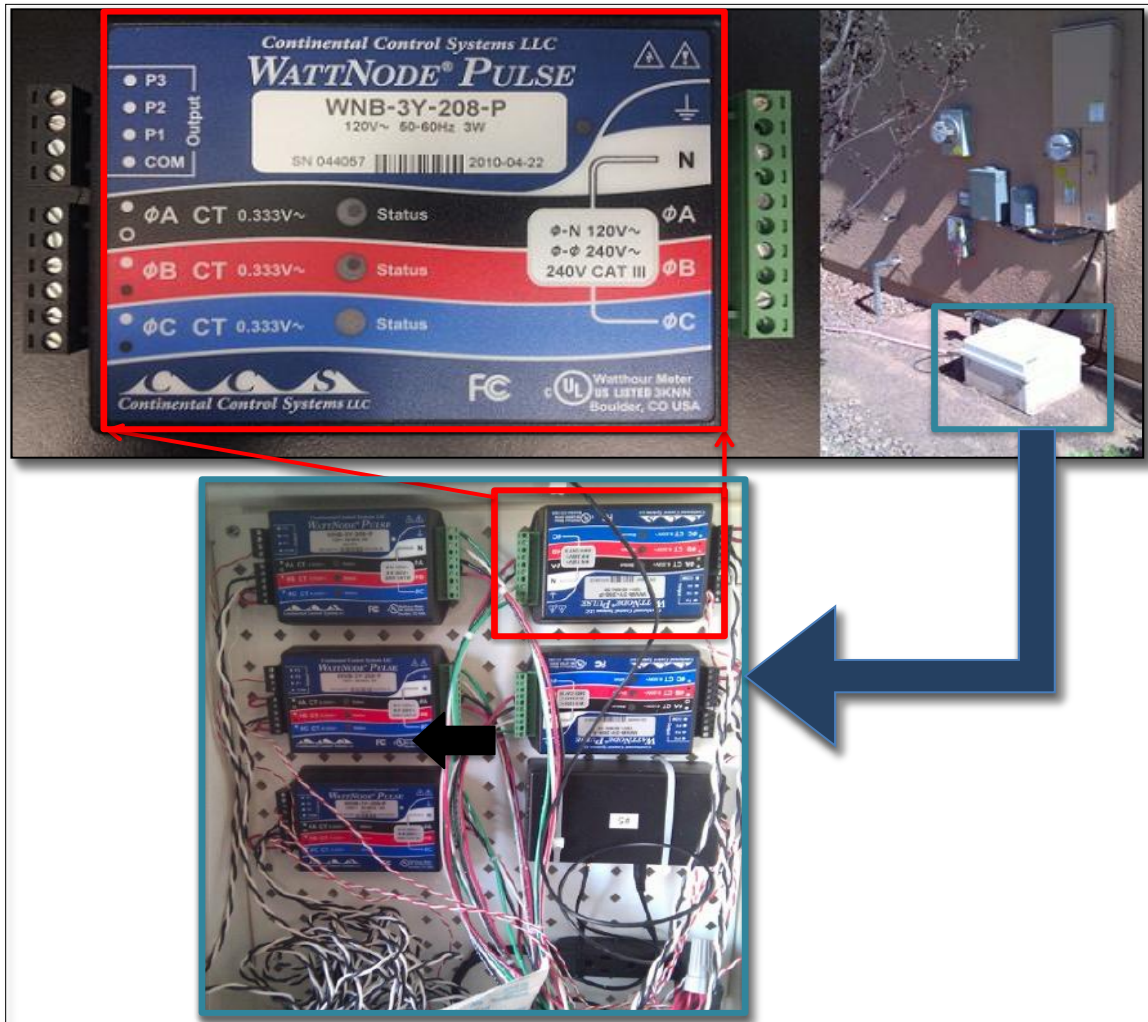
Figure 19 – WattNode model WNB-3Y-208-P and Installed Project Box.
