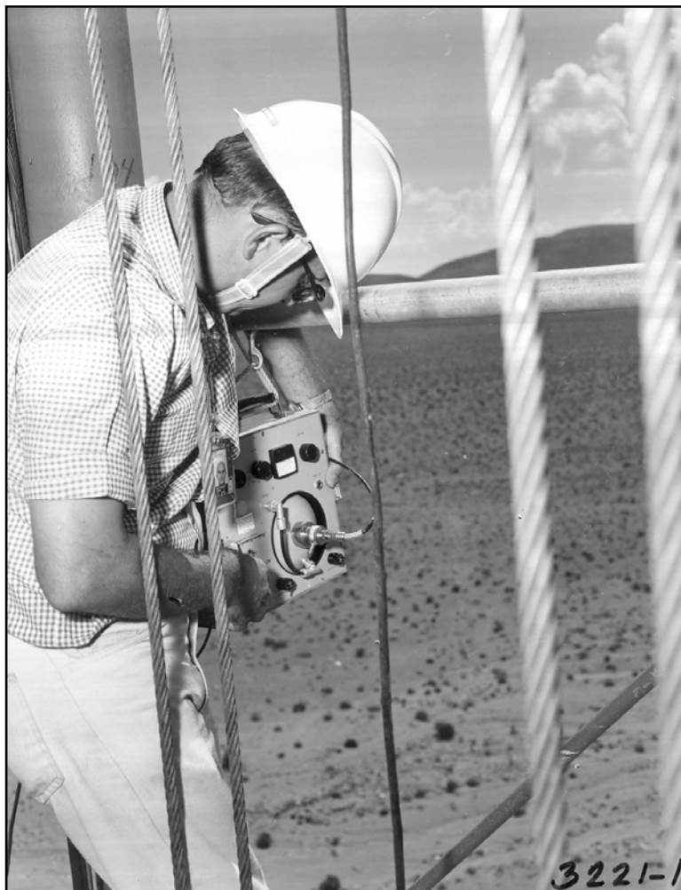
Photo 85. Technician rigging BREN Tower with instrumentation for the sonic boom tests. Photo taken August 26, 1970 (Photo 3221-16 on file at NNSA/NSO Nuclear Testing Archive).
