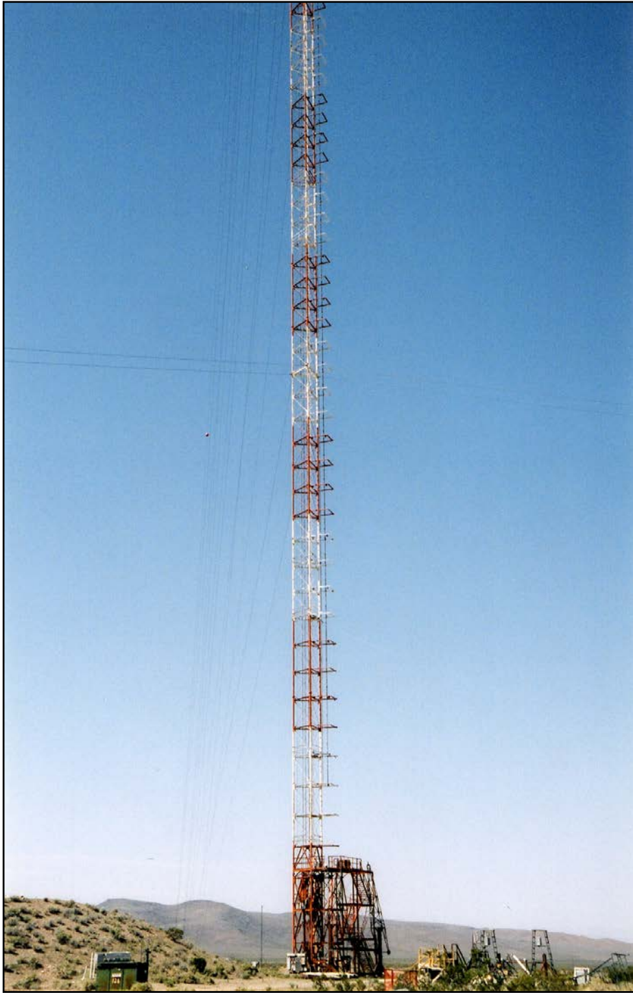
Photo 5. The BREN Tower today. Only the lower 300 ft of the tower and the main work platform are visible in this photo taken by DRI in June 2004. The Control Bunker is to the left. Discarded equipment and debris from the various experiments conducted at this location from 1966 through the mid 1990s appears at the lower right. View is to the southwest (on file at NNSA/NSO Curation Facility).
