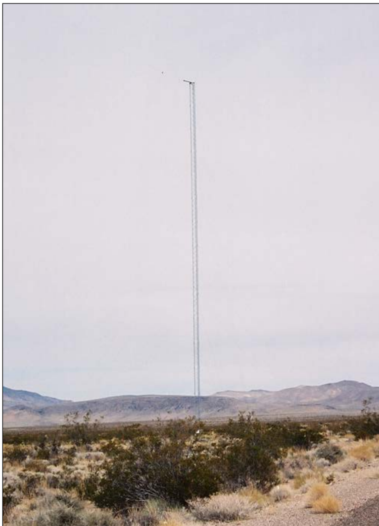
Photo 58. Tower 3.2 used in Operation HENRE Program 3. The pulley and cable system used to suspend the instrumentation for the experiments is visible at the top of the 150 ft tower. View is to the northeast. Photo taken by DRI on November 1, 2006 (on file at NNSA/NSO Curation Facility).
