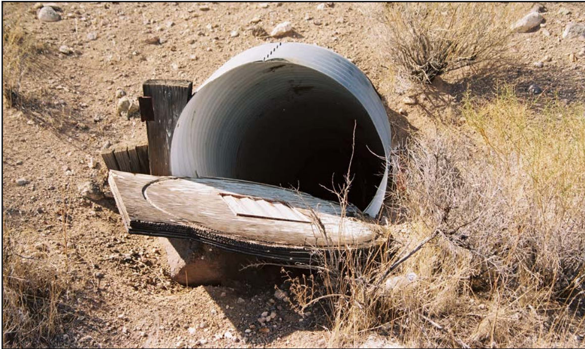
Photo 22. Detail of entrance to the underground civil defense shelter. Wooden door has fallen open since the June 2004 field inspection. View down and to the west. Photo taken by DRI on November 1, 2006 (on file at NNSA/NSO Curation Facility).
