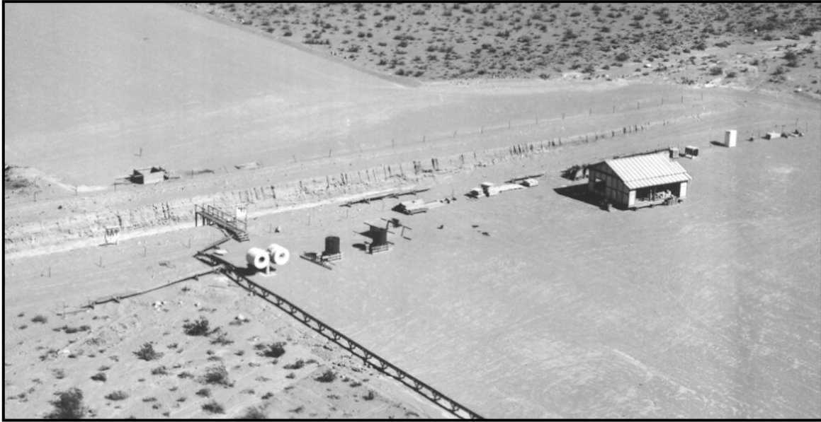
Photo 47. A 1966 overview showing, from left to right, a cable trough and stairs leading to recording trailers in the revetment, a pair of turret-mounted collimators, a pair of platform mounted collimators, stacks of extra transite panels, pipe and supplies, the analog Japanese House, and a porta potty. The crates of authentic Japanese building materials are partially visible behind the Japanese House as is one of the concrete prisms. The trailer revetment, surrounded by a T-post fence extends across the photo behind the house. The cable trough and stairs have been removed and the paired collimator was replaced by an instrument tower for later (post-1970) experimental programs. View is to the northeast (Photo 2581-14 on file at NNSA/NSO Nuclear Testing Archive).
