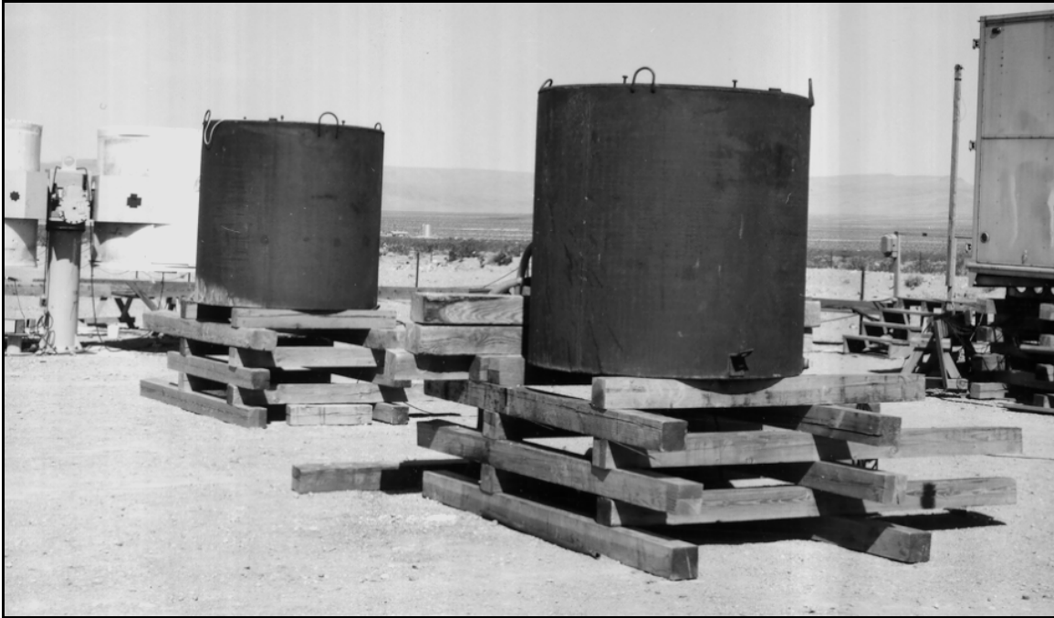
Photo 37. August 1967 photograph of the pair of platform mounted collimators located at 2,250 ft from BREN Tower. A pair of the insulated turret-mounted collimators is in the background at the left and the corner of an Oak Ridge National Laboratory Radiation Dosimetry Health Physics Division support trailer appears on the right. View is to the northwest (Photo 2518-5 on file at NNSA/NSO Nuclear Testing Archive).
