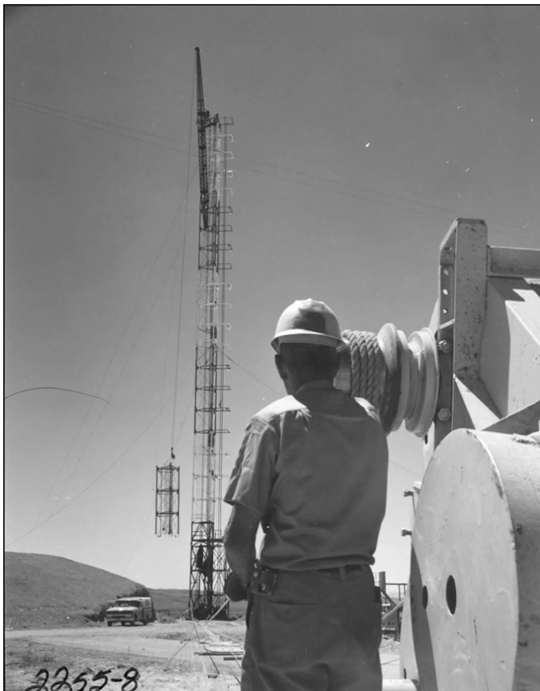
Photo 2. BREN Tower being reassembled at NTS Area 25, May 12, 1966. Temporary guy wires stabilize the tower during construction. The earth mound covering the Control Bunker appears on the left behind the truck. View is to the west (Photo 2255-8 on file at NNSA/NSO Nuclear Testing Archive).
