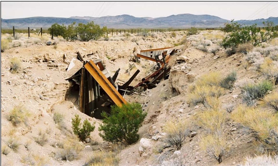
Photo 77. The covered trailer revetment located 750 ft from the base of BREN Tower was used to shelter the recording trailers for Operation HENRE experimental Programs 2 and 9. The wood and metal cover has collapsed. View is to the northeast. Photo taken by DRI on November 01, 2006 (on file at NNSA/NSO Curation Facility).
