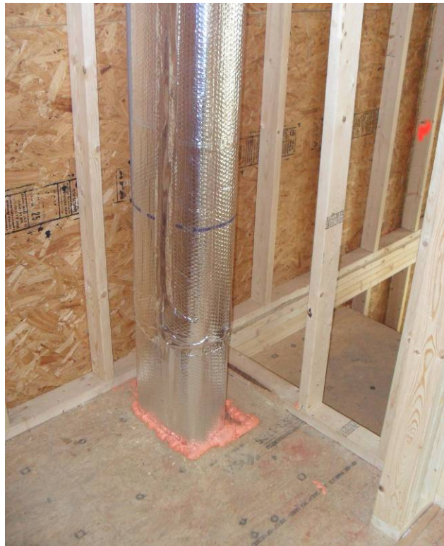
Figure 11. Duct during framing
