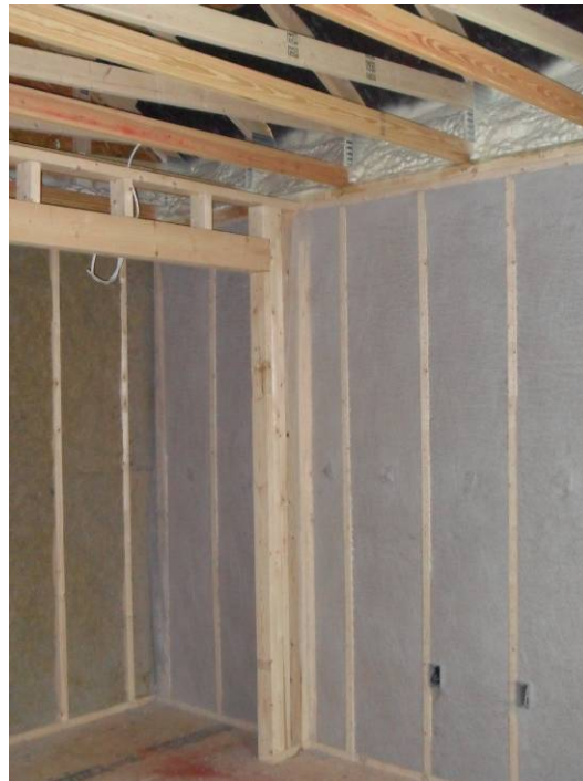
Figure 7. Above-grade walls with dense pack cellulose insulation
