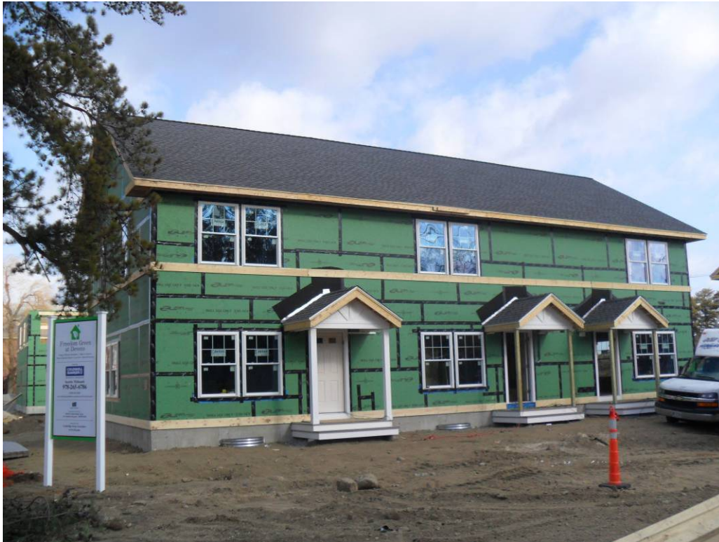
Figure 6. Triplex during construction
