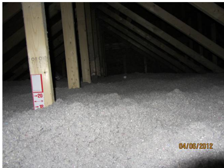
Figure 9. Attic insulation
