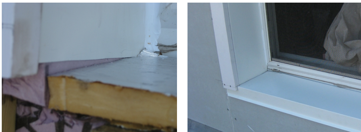
Figure 42. (L) Insulation return at the jamb installed before the insulation return at the sill. Note also that the sill flashing membrane does not extend over the outer face of the insulating sheathing. This was later corrected. (R) Sill trim installed after the jamb return trim. Sill extensions are actually cut around the jamb trim. Note that the window sill trim has a kick-out to direct water away from the face of the building.
