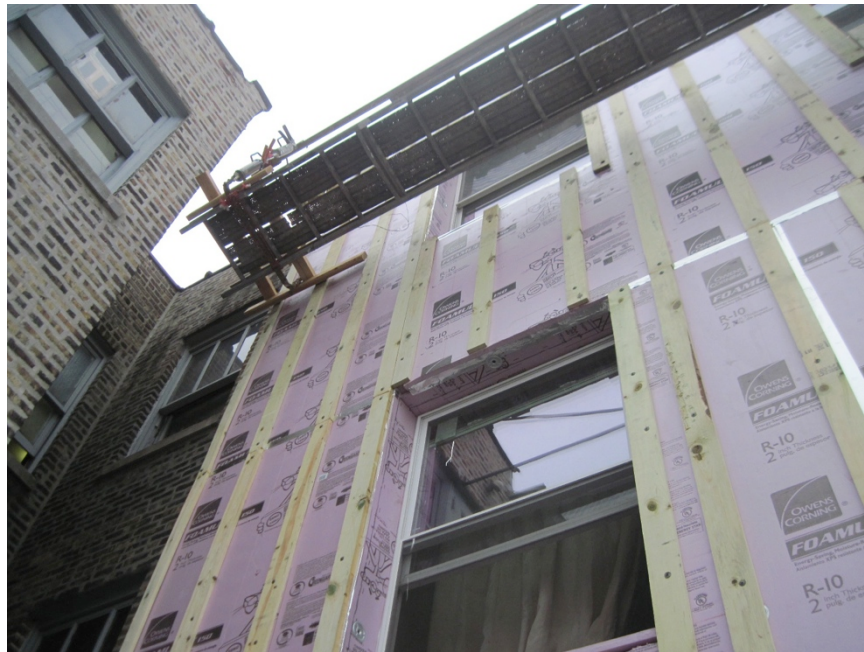
Figure 23. Wood strapping installed in vertical orientation only over face of insulating sheathing (Credit: Scott Sanders, CEDA)
