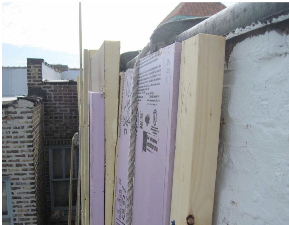
Figure 26. Beveled roof insulation used to true new cladding attachment at top of wall. Note that fasteners are left loose at the time of this photo. (Credit: Scott Sanders, CEDA)
