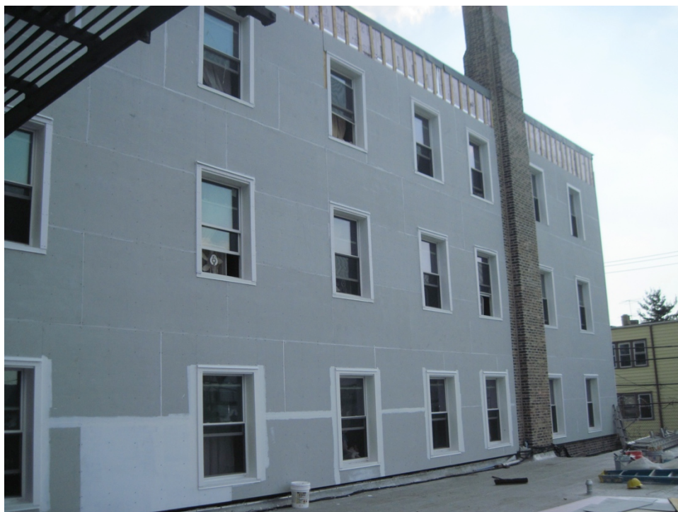
Figure 51. Caulked butt joints between 4 × 8 panels
