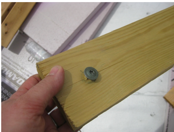
Figure 24. (L) Wood strapping with fastener used for attachment through rigid foam insulation to 2 × 4 framing; (R) longer size fasteners used to attach strapping through thicker rigid foam insulation layer at parapet
