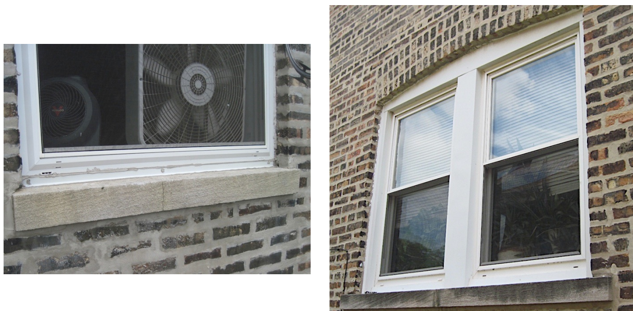
Figure 36. (L) Window set directly in masonry opening at the larger building; (R) windows set in metal-clad trim/frame surround at the two-family building (Credit: Scott Sanders, CEDA)
