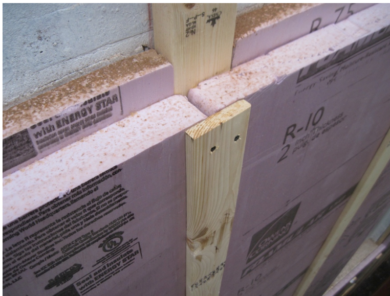
Figure 22. Offset of seams in successive layers of insulating sheathing. Offset for vertical seam is limited by the size of insulation boards and the spacing of framing. (Credit: Scott Sanders, CEDA)
