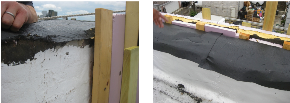
Figure 30. (L) Transition membrane not connected to elastomeric coating at face of wall; (R) transition membrane not adhered to roof membrane at inside face of parapet
