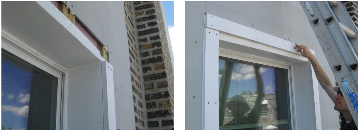
Figure 45. (L) Window head return trim sloping toward the window; (R) CEDA personnel demonstrating the reconfiguration of the window head return trim
