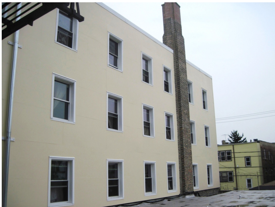
Figure 48. Finished side of the larger building
