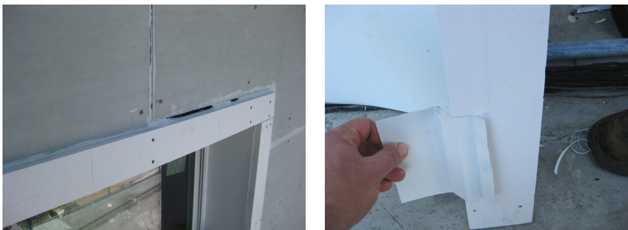
Figure 46. (L) Window head casing with no drip cap and sealant gaps; (R) Contractor project manager reviewing the drip cap flashing with the crew
