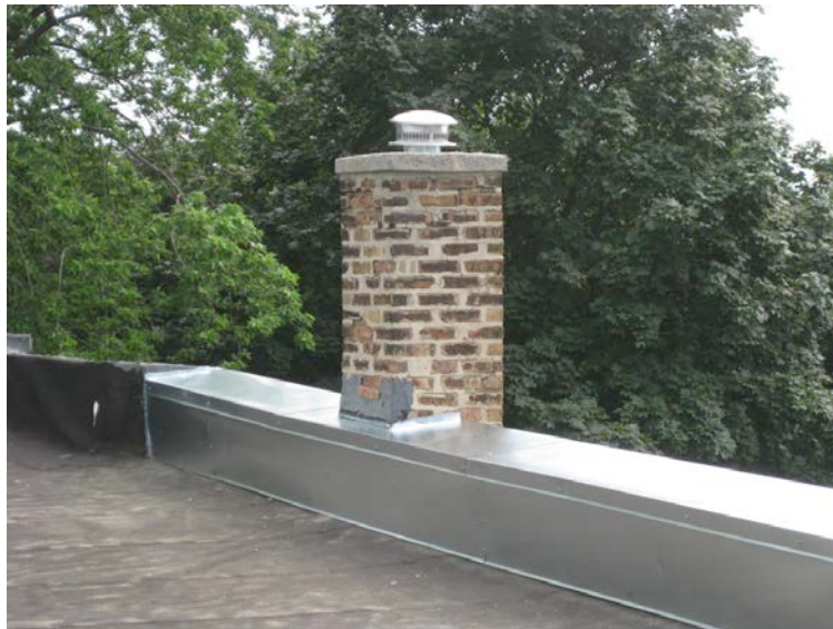
Figure 29. Finished parapet cover at two-family building
