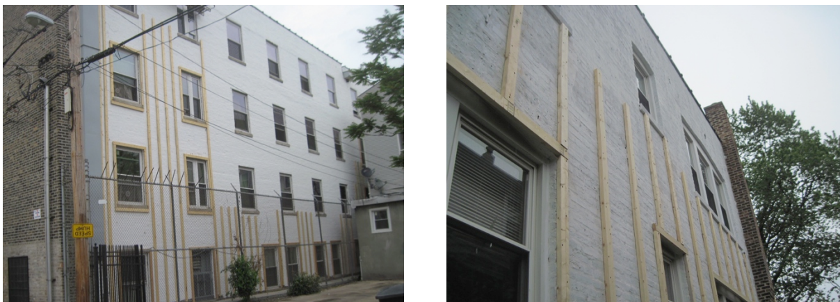
Figure 19. (L) Framing installed at in a vertical orientation only in the field of the wall. Each window opening is picture framed with the framing material. (R) Framing installed against masonry at two-family building with horizontal framing at top of window openings but in a vertical orientation elsewhere. (Credit: Scott Sanders, CEDA)
